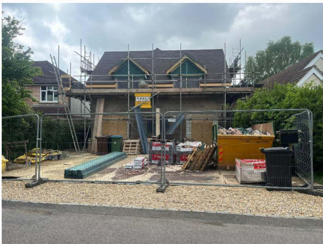
[Photo 15 – Property under construction (front view): active redevelopment within the street]
