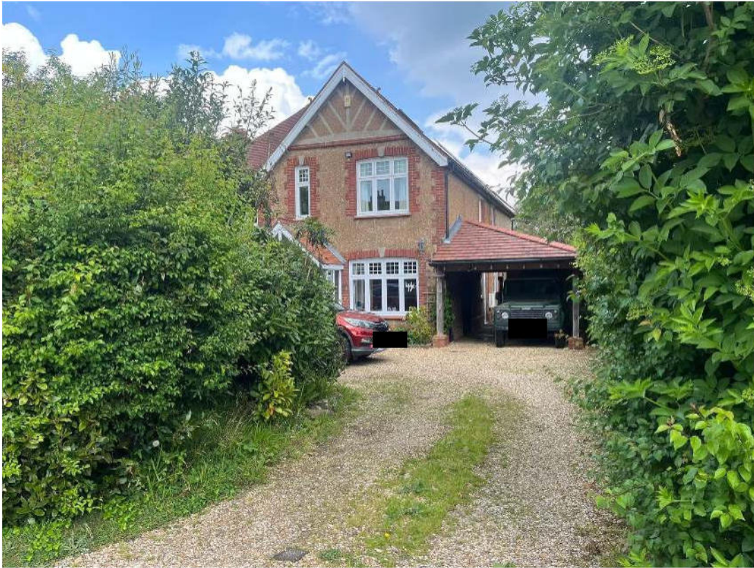
[Photo 3 – No. 44 (adjacent house): differing scale and architectural form]
