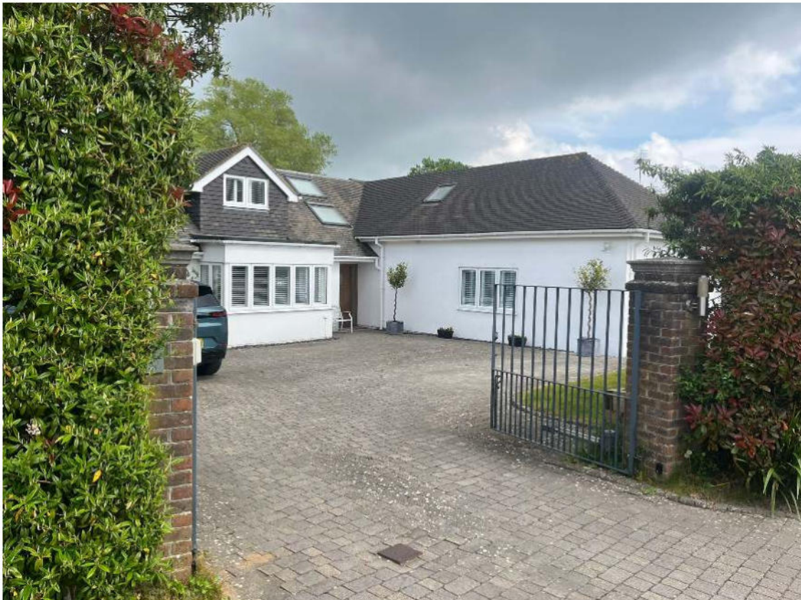
[Photo 6 – No. 41: side and main building showing scale and siting]
