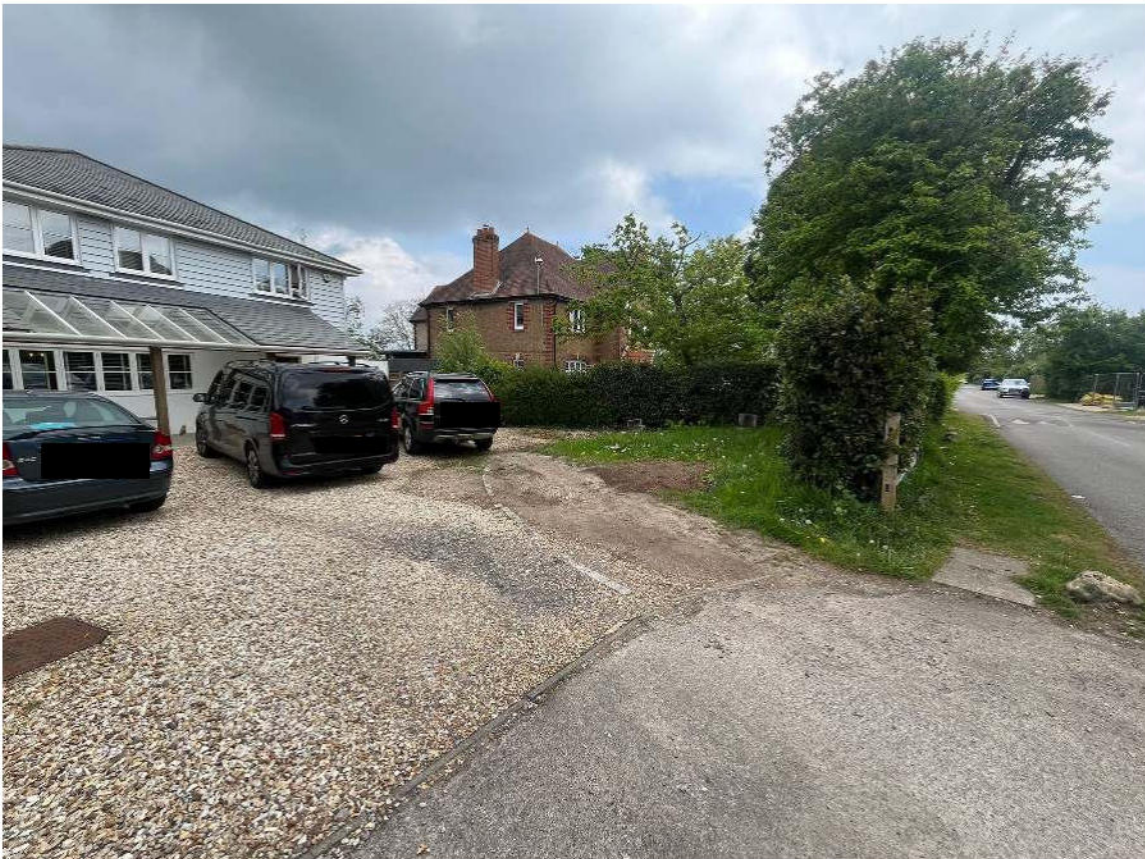
[Photo 1 – Front of Wycombe, 43 Elm Grove: view of the existing dwelling and frontage]
