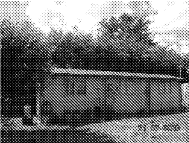
Photo 10: Modern cabin to be retained
