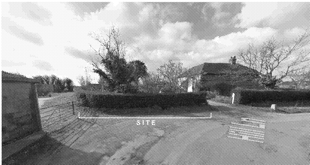
Front of site and 33, Hill Lane
