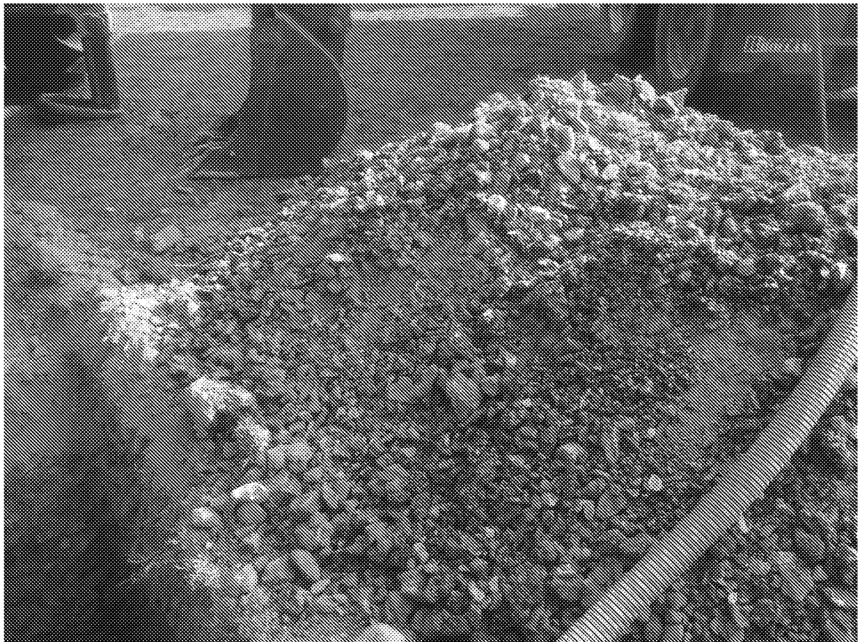
PLATE 16 – Trial pit TP4 arisings
