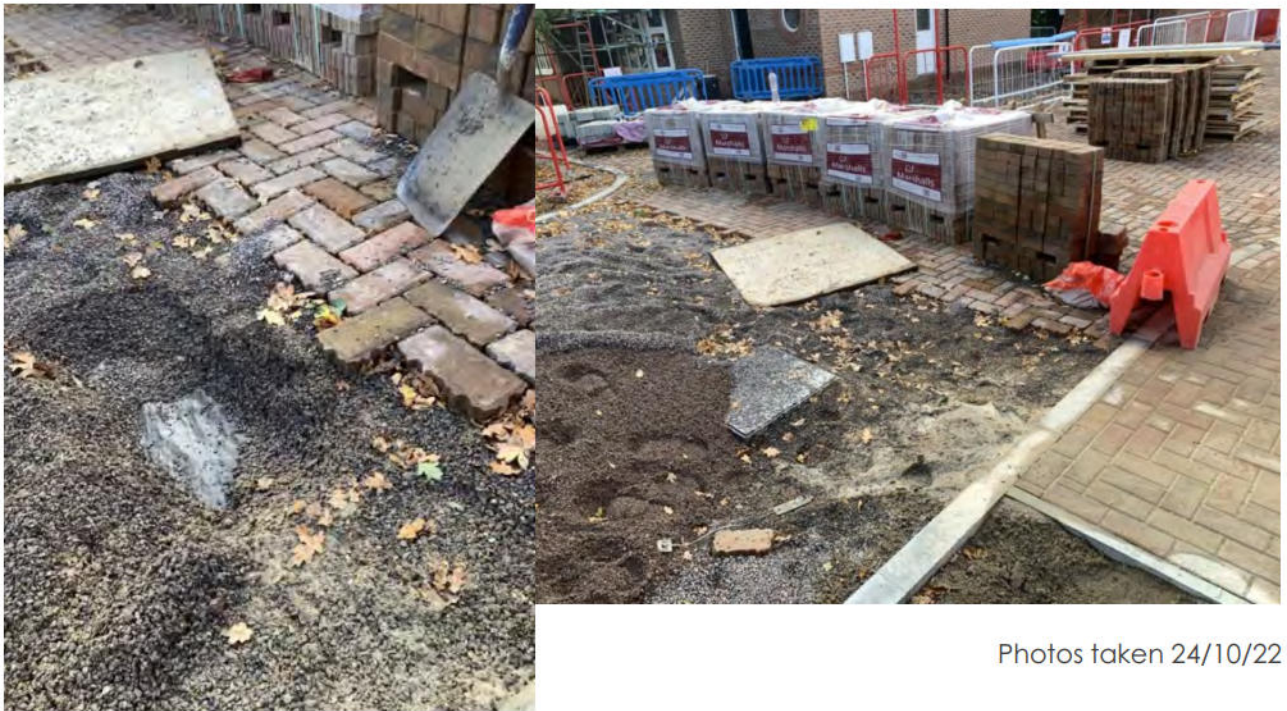
Photo 4 - Zone 5 Permeable paving mid construction, shows paving blocks on grit bed over terram
