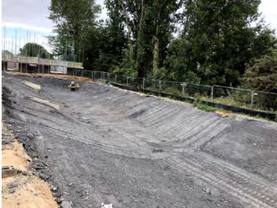
Photo 5 - Compaction of blue clay liner
