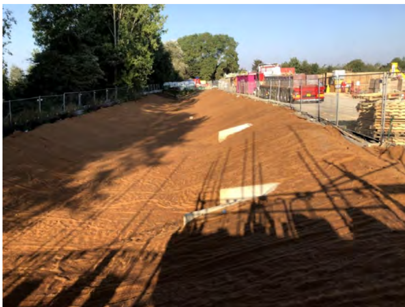
Photo 10 - Finished bio-degradable erosion mat looking west
