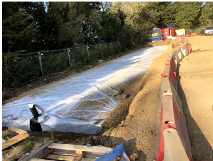
Photo 18- Backfill of attenuation tank looking west
