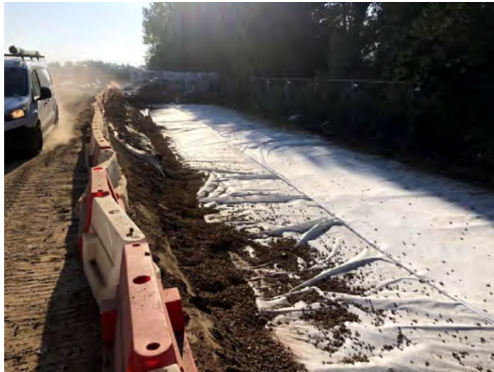
Photo 17 - Backfill of attenuation tank looking east
