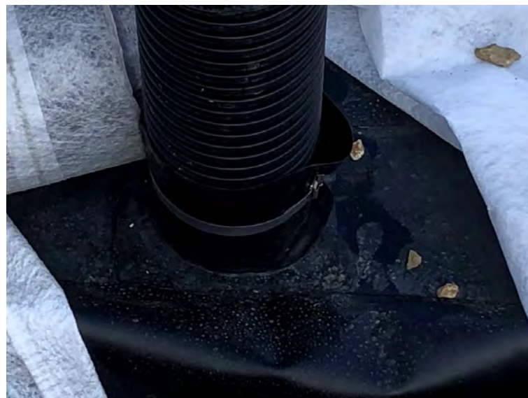
Photo 16 - Shows welded geo-membrane around air vent
