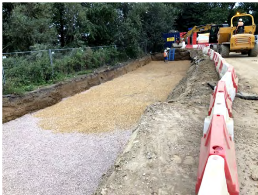
Photo 12 - Shingle base complete
