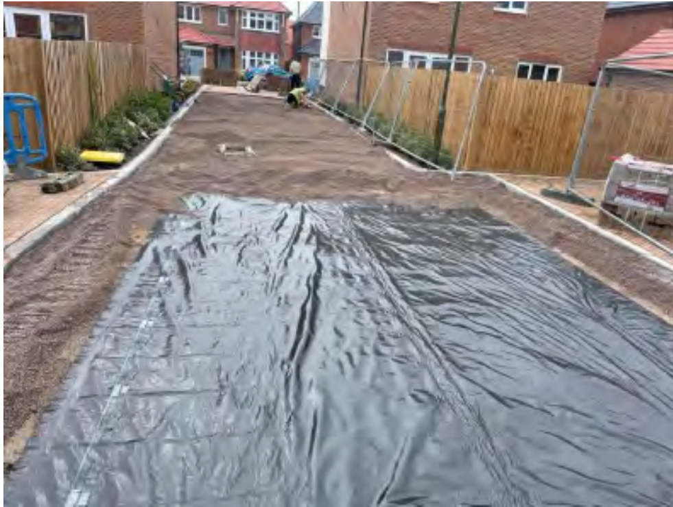
Photo 2 – Laying of Terram and 6mm chip bed (Photo taken 30/06/22)
