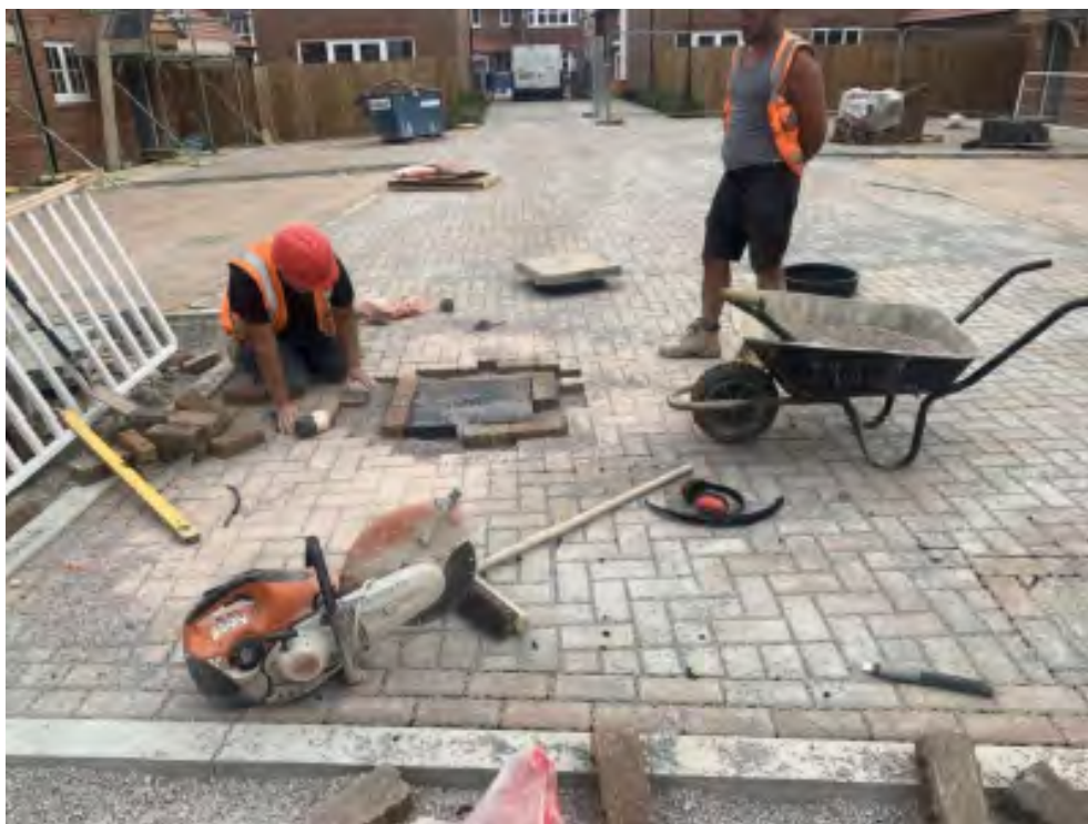
Photo 3 – Laying 60mm permeable blocks zone 3 and 4 (Photo taken 6/07/22)
