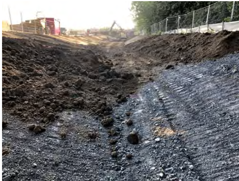
Photo 7 - Placing 150mm topsoil layer over clay
