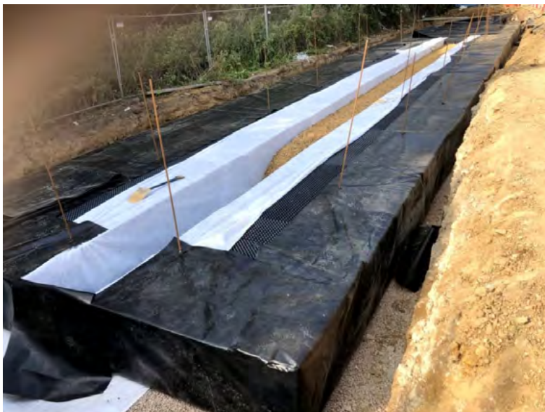
Box 14 - Shows central perforated pipe wrapped in geotextile back filled with fines free shingle crates both sides looking west
