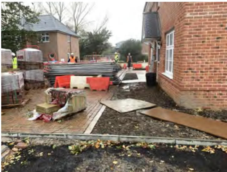
Photo 5 - Permeable Paving complete Zone 5 (Picture taken 1/11/22)
