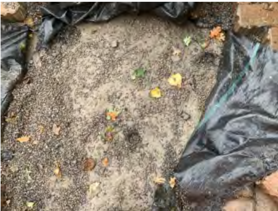
Photo 1 - Drainage holes drilled through asphalt base ( Zone 5 also shows terram layer )
