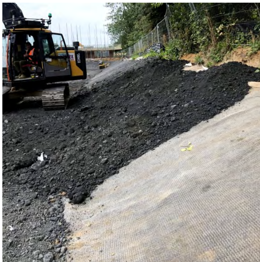
Photo 4 - Shaping southern bank to achieve 1 in 3 slope
