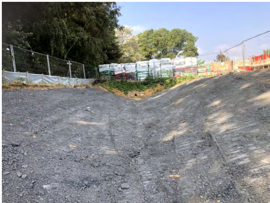
Photo 6 - Blue clay liner looking west towards inlet pipe
