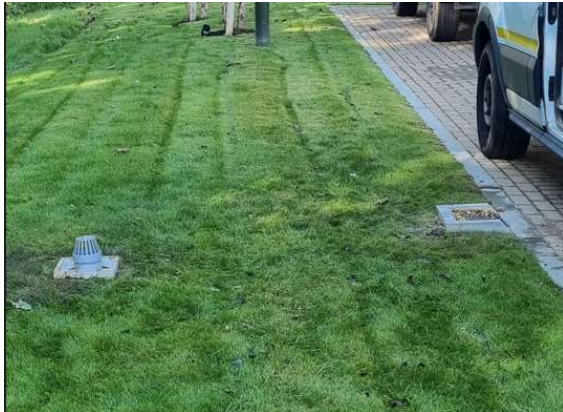
28-09-2024 Vent pipe and rodding eye from attenuation tank.
