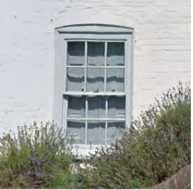
Painted window frames
