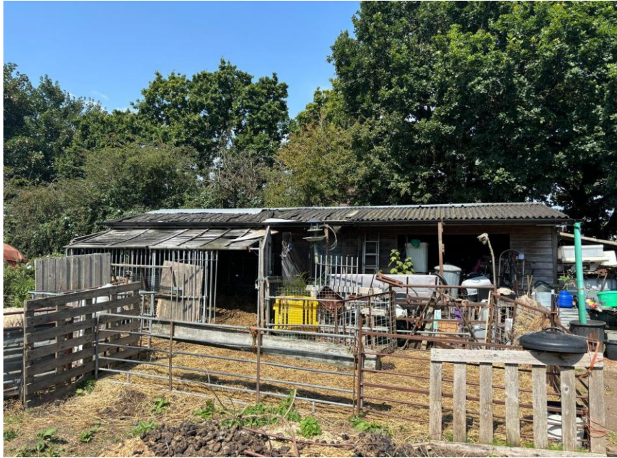
Figure 7. The southern elevation of the building (taken August, 2024).
