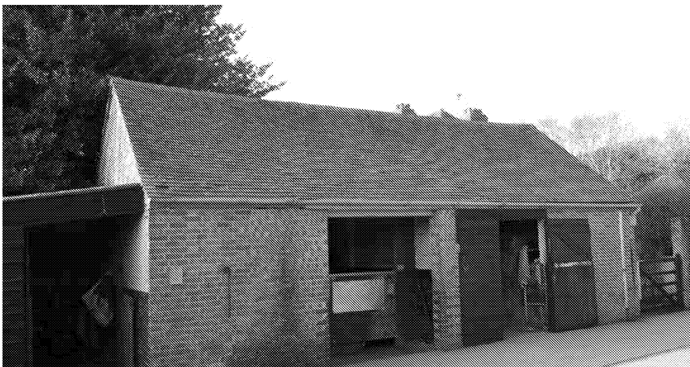
Photograph No. 24 - The traditional stable Building B6.
