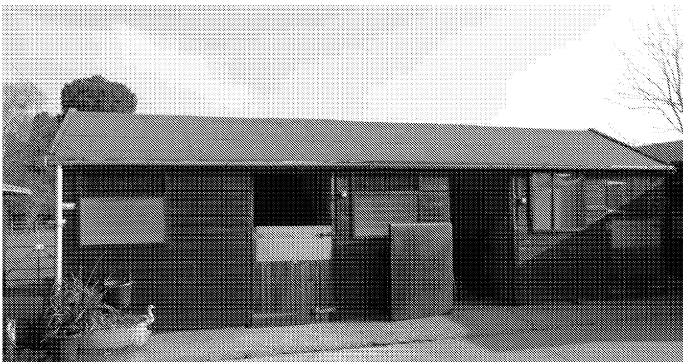
Photograph No. 26 - The stable Building B8.
