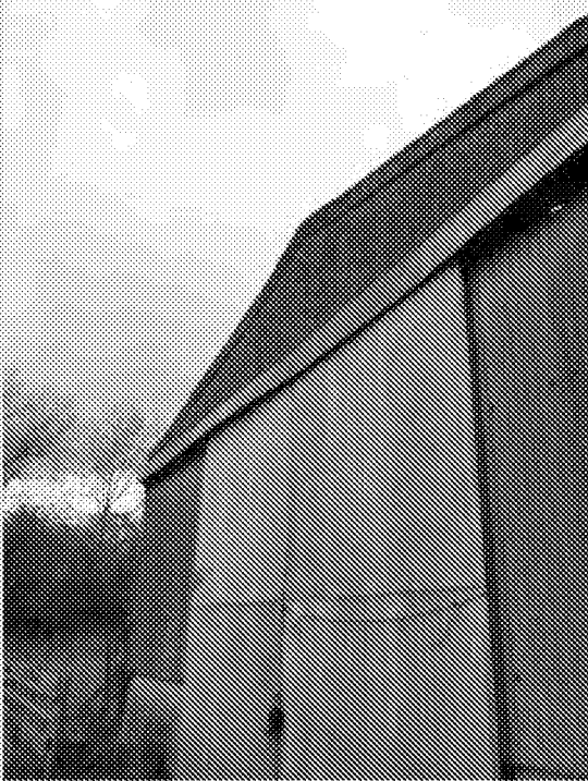
Photo 1. Southern aspect of building B2
