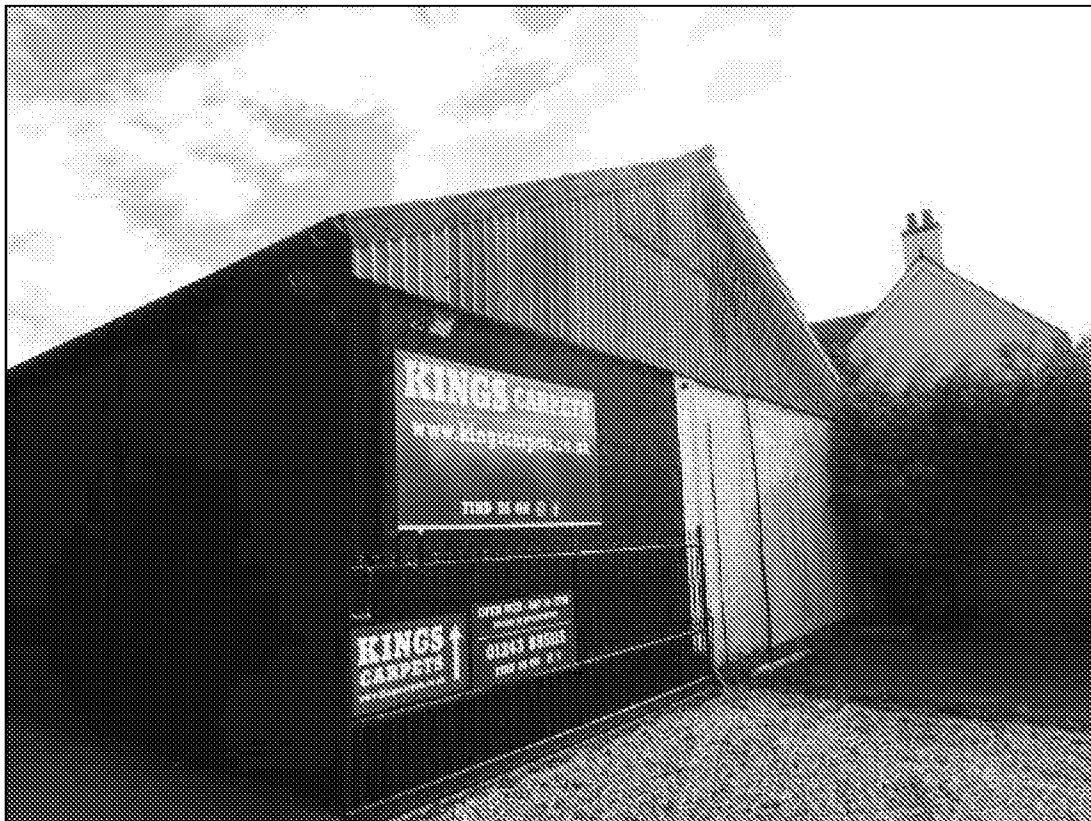
Commercial Building A.
