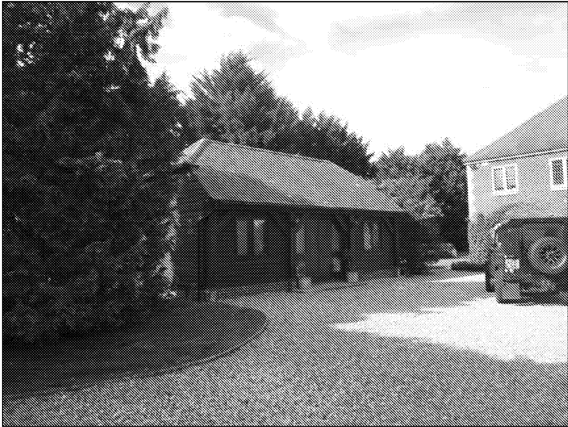
The existing garage.
