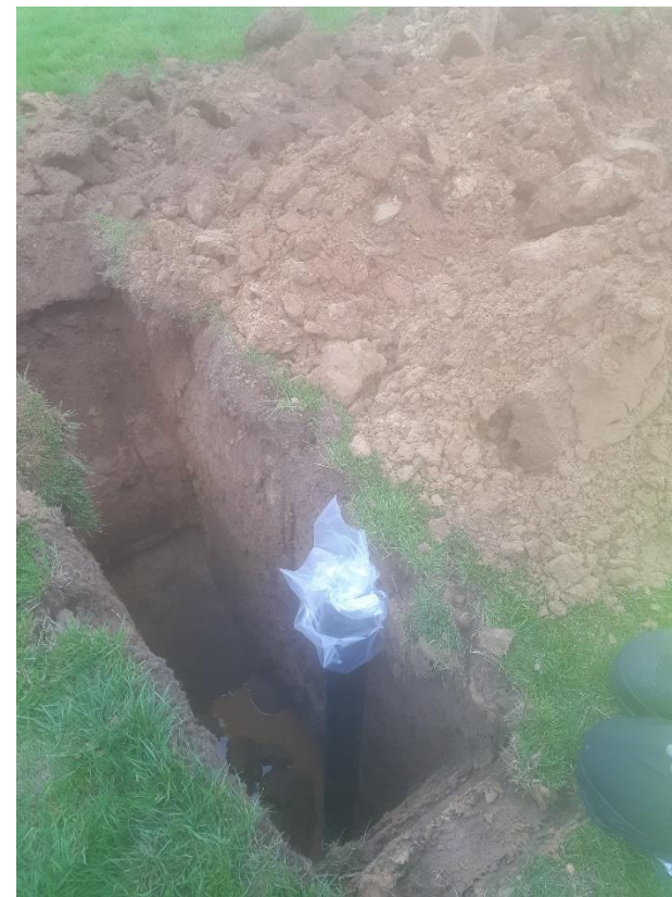
Plate 16: TP49 soakage pit before gravel fill
