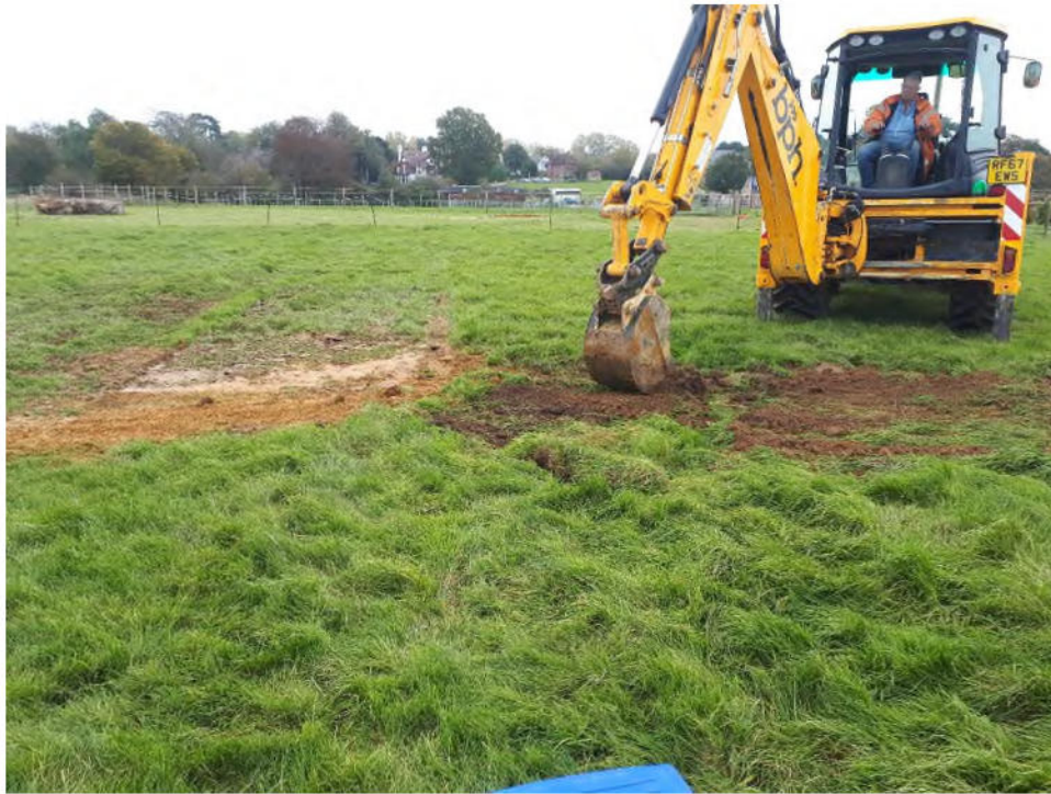
Plate 7: TP47 (right) and TP47a (left) after backfill
