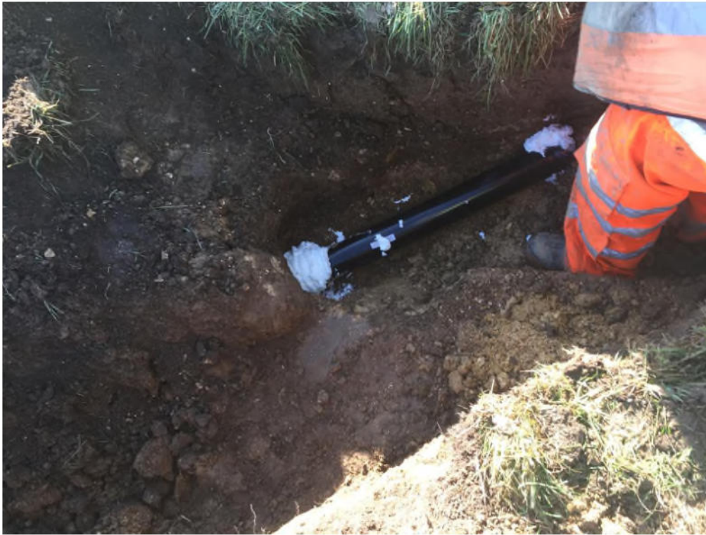
Plate 9: Land drain repair
