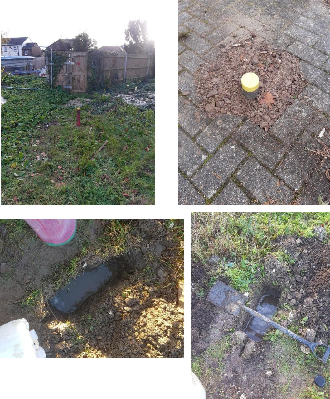
Fig 3. Groundwater Monitoring Well locations and soakaway test photographs
