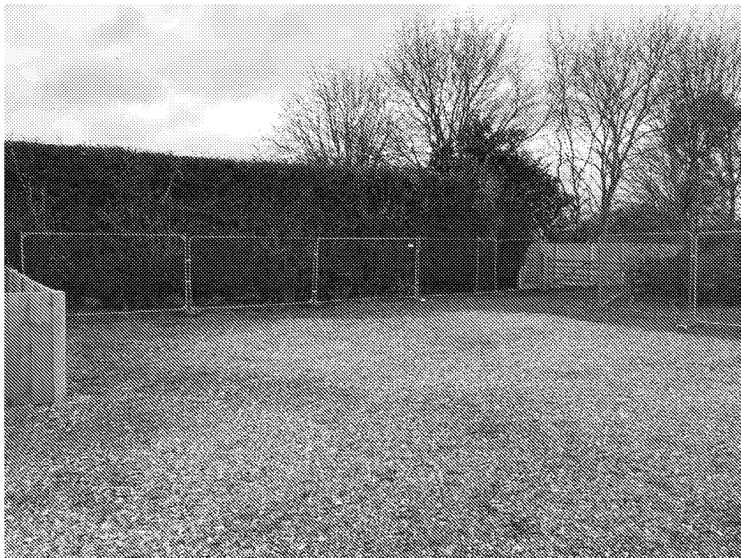
The protective fencing in place to protect Hedge 1 - conifers.
