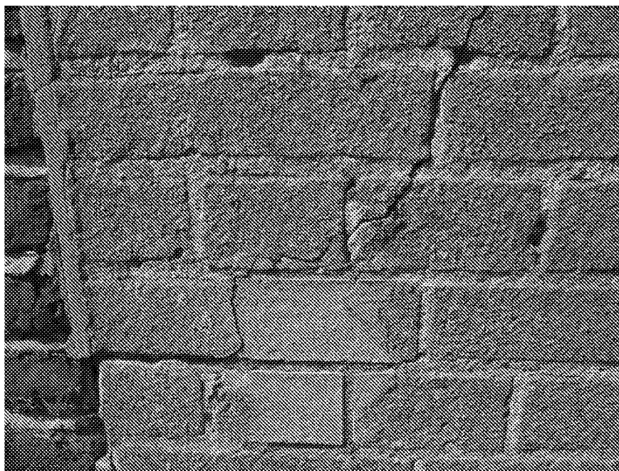
Figure 4 - Refaced brick with render and pointing over existing.
