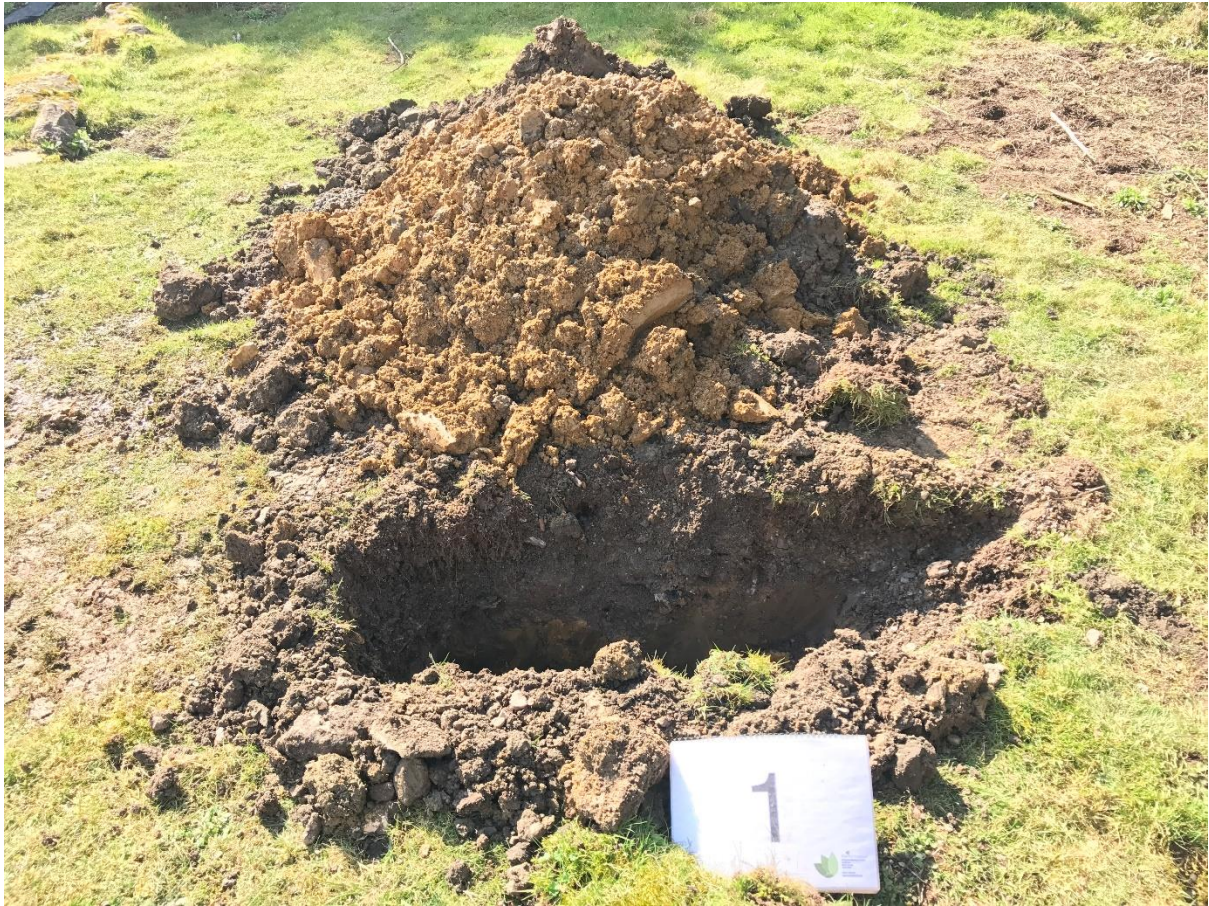
Record Photo of Trial Pit 1
