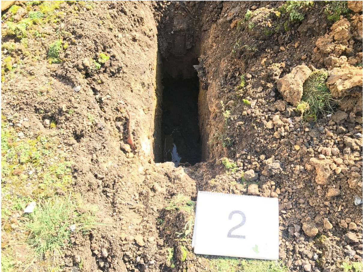
Record Photo of Trial Pit 2
