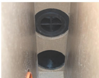
View of foul air trap before installation
