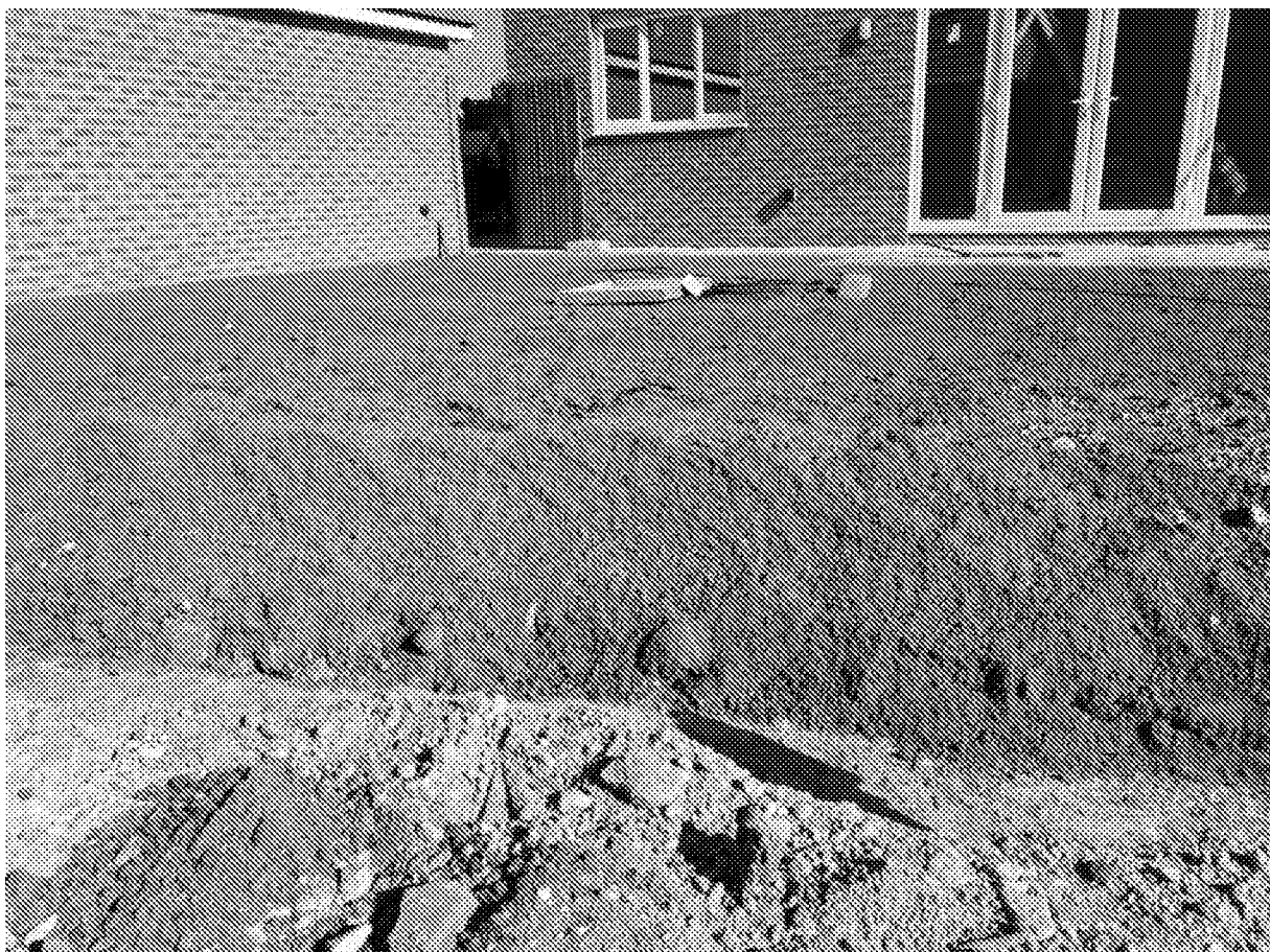
Plot 49 – edge of placed capping material (adjacent to garden wall which is to be constructed)
