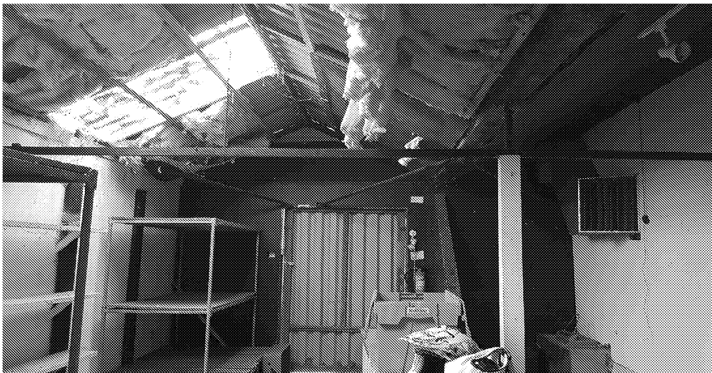
Photograph No. 7 - Interior view of Building B3.
