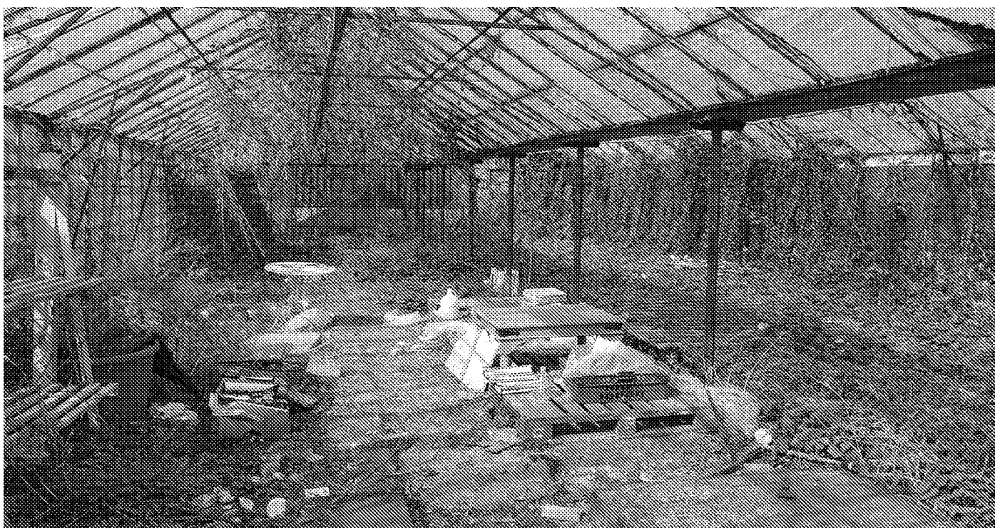
Photograph No. 6 - Interior view of Building B2.
