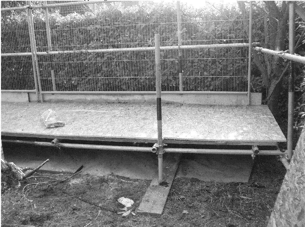
Photo 2 Scaffold framework supporting wooden boards
