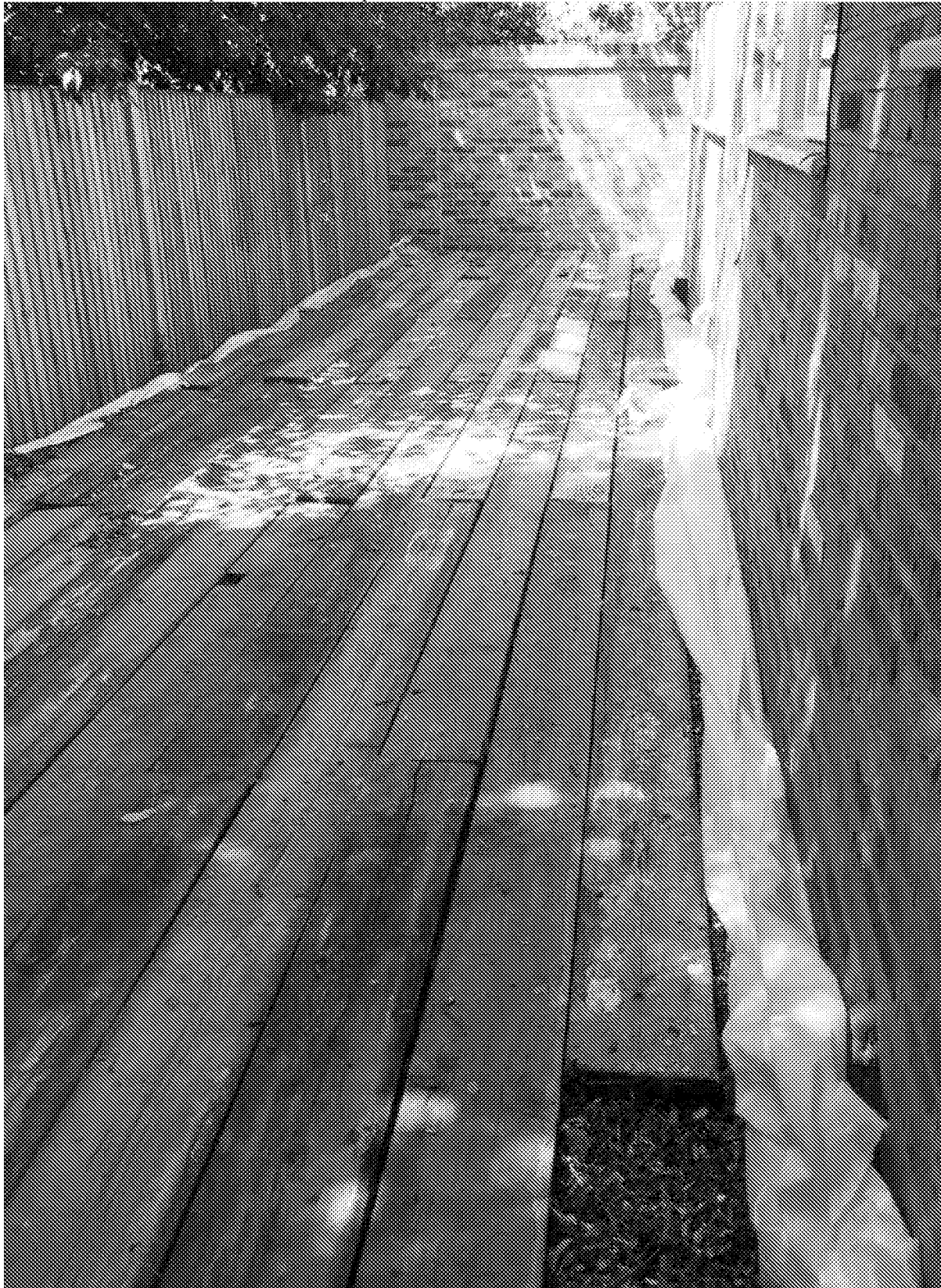
Photo 1. Scaffold boards placed on woodchip
