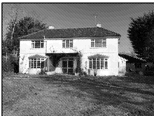
Figure 8 – south-western elevation of the main section of the house
