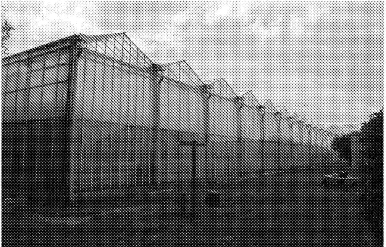
Landscape Character Photo D: Commercial Horticultural Buildings
