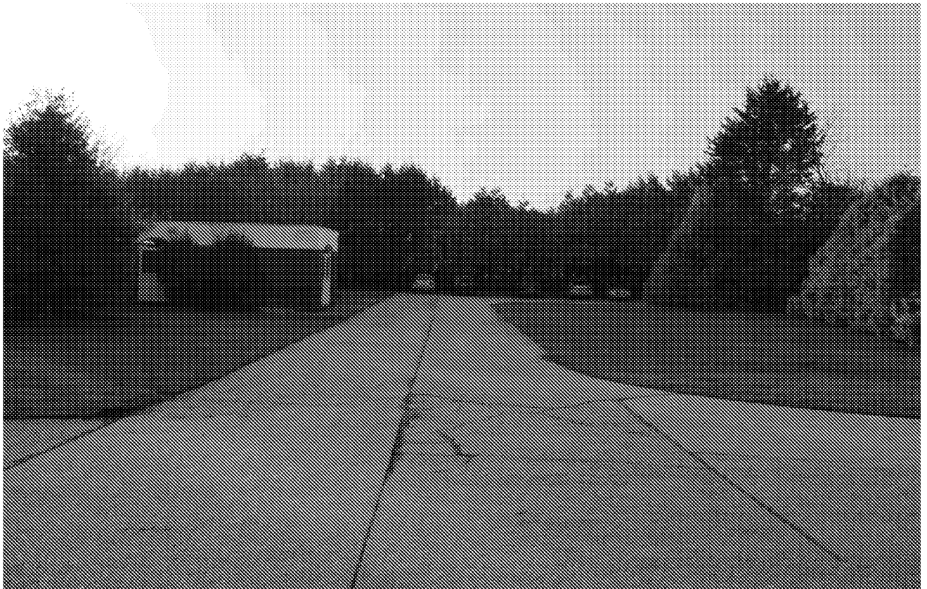
Viewpoint No 9: Eastern Boundary Looking West
