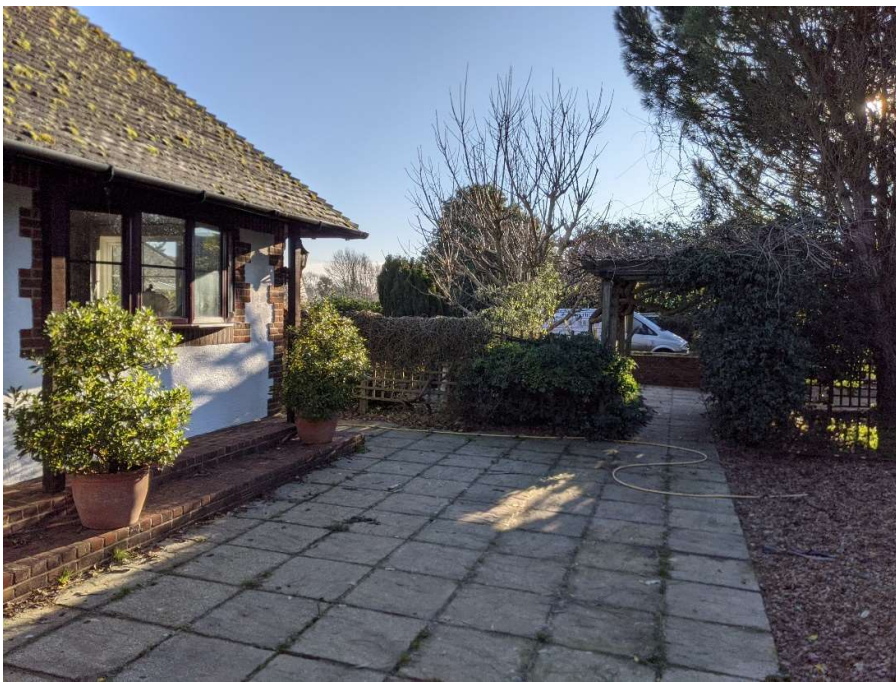
View of the site and ex garage from the north adjacent to The Cottage.
