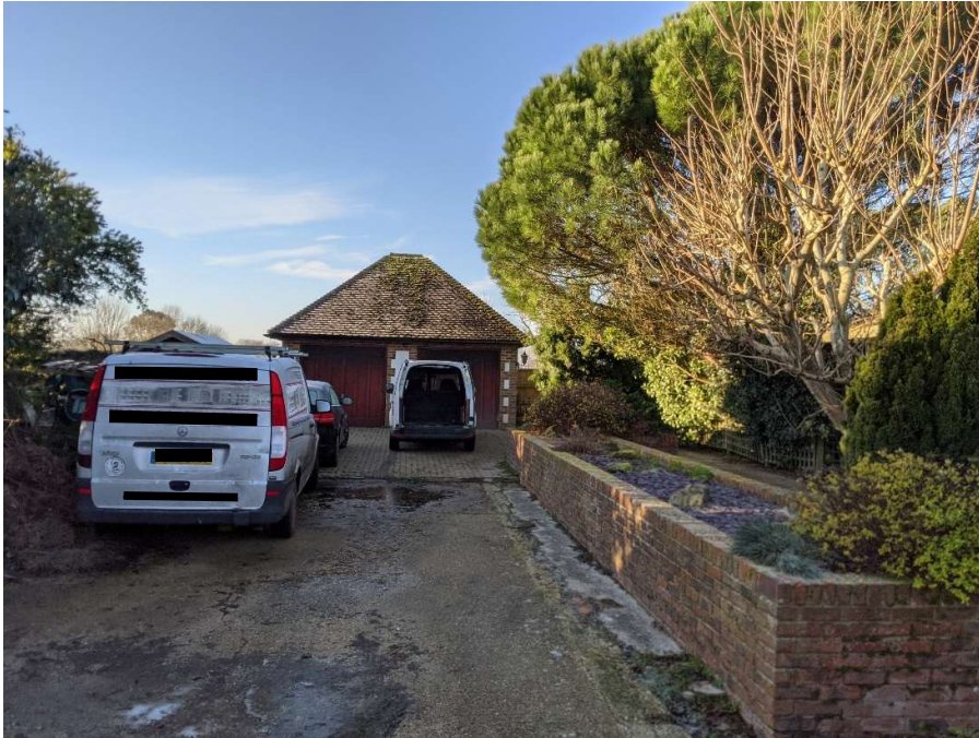
The application site – Existing garage to be part retained.
