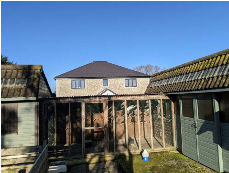
View of The Fallows (recent detached two storey dwelling) to the rear of The Cottage.
