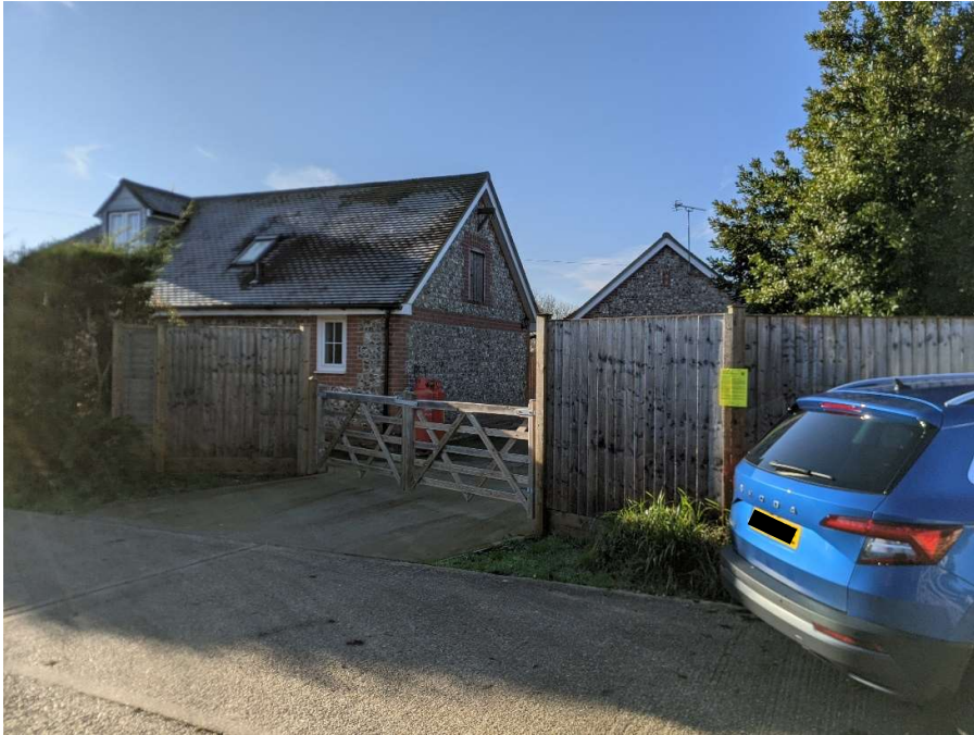
Drive to Crabapple Cottage and Russet Cottage at the head of the Access Road.
