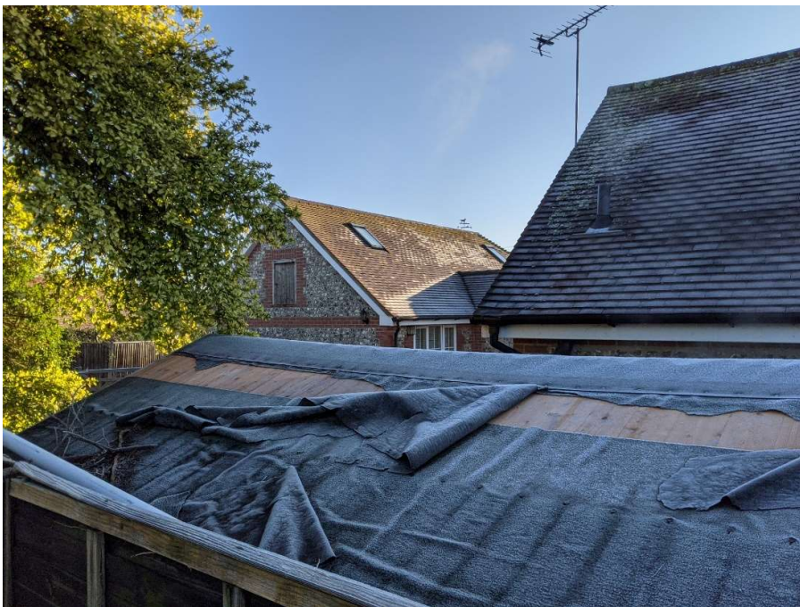
Carbapple Cottage to the rear (LH) and Russet Cottage to the front (RH) & the garden shed serving Russet Cottage adjacent to the ex fence.
