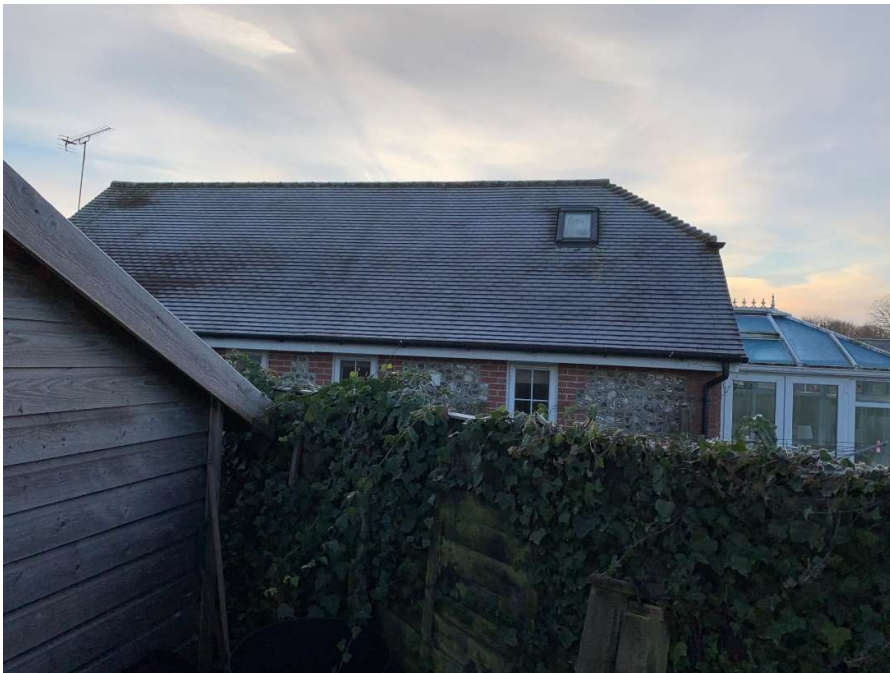
Russet Cottage side elevation facing the site.
