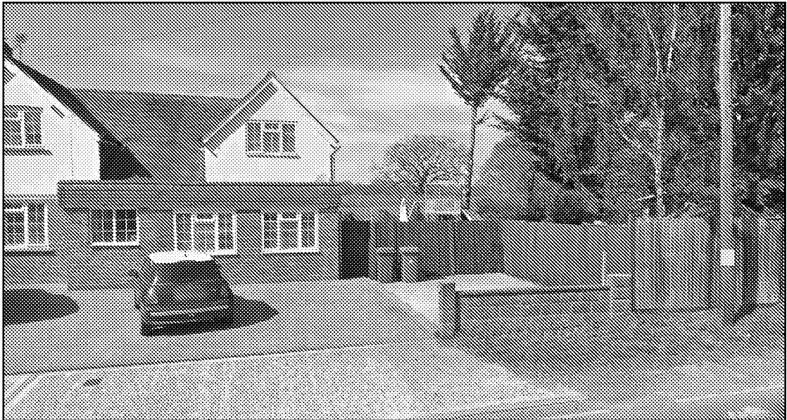
Figure 9 Gap in roadside screening 1
