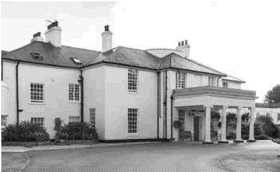
Westergate House - Grade II
