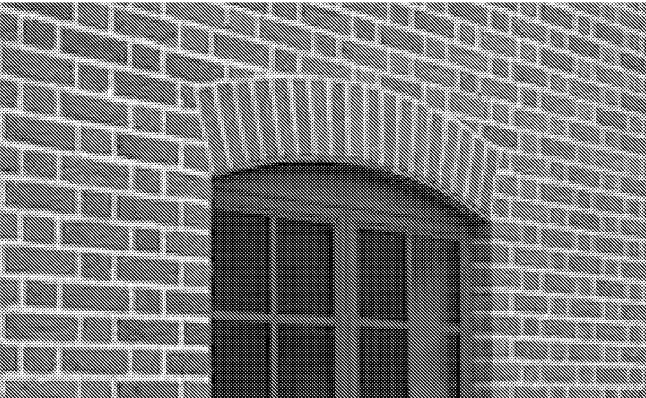
Brick header detail
