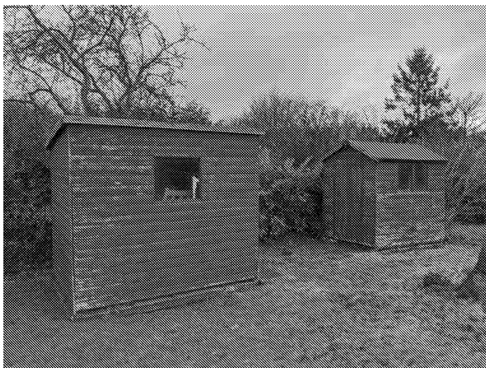
Photograph No. 4 - View of the sheds (Buildings B1 and B2) which offer negligible bat roost potential.
