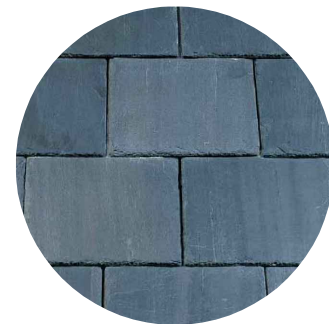
Roof - Slate Tile
