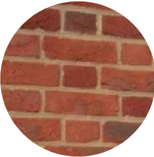
Upper Walls/Lower Walls - Brick
