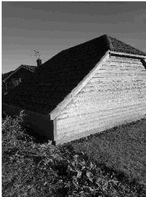
Photo 17: Southern elevation of B4
