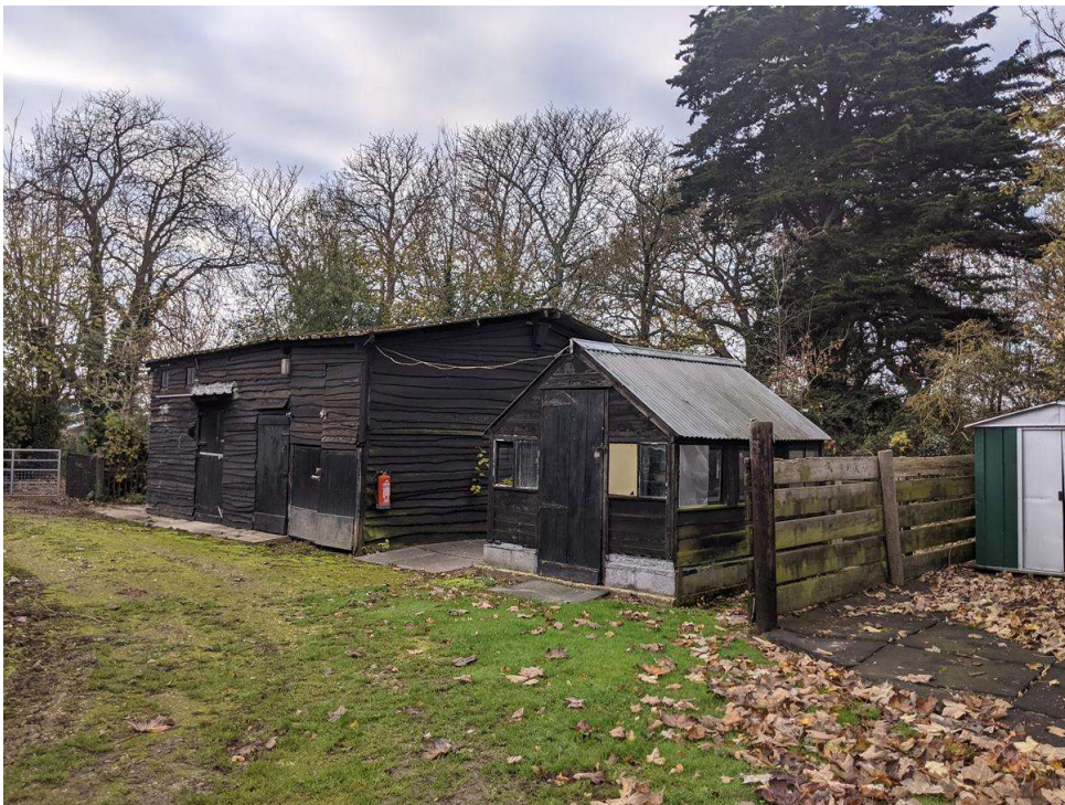
Photograph 4 – Buildings B02, B03, B04 (Left to right). Bat box visible to centre of gable end of B02 just beneath ridge.
