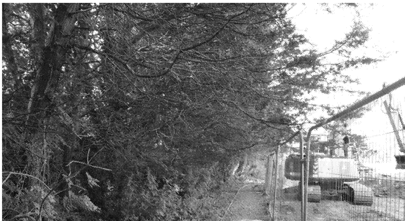
Photograph No. 10 - Footpath link from the south-eastern edge of the site area - low bare canopies of the underplanted Leyland Cypress trees looking westward.
