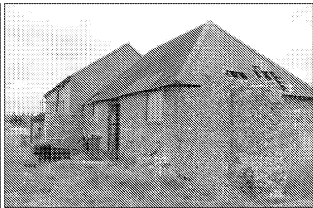
Plate 8. Surviving barn structure, looking north-west.
