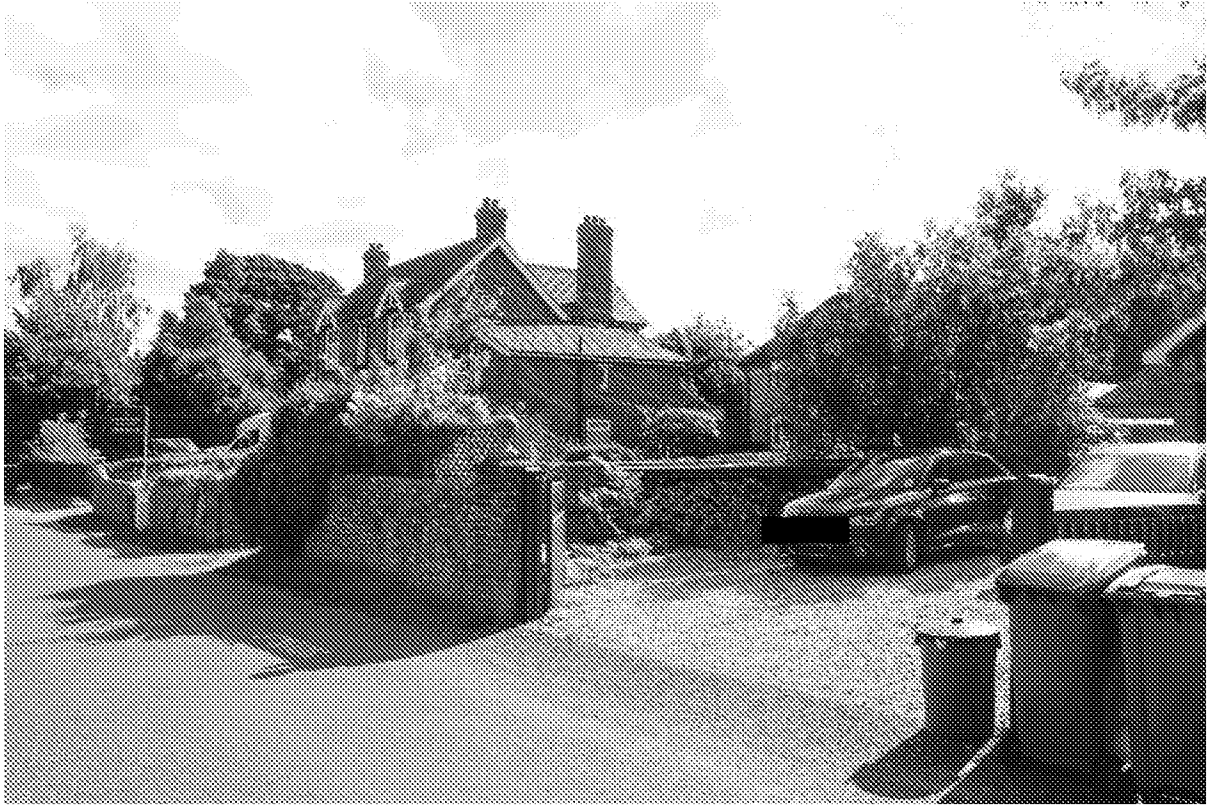
Image EDP 22: Representative view of Curacoa looking north-east from Church Lane and showing its position in the streetscene and modest proportions in direct comparison with the adjacent 20 th century property on its north-eastern flank.
