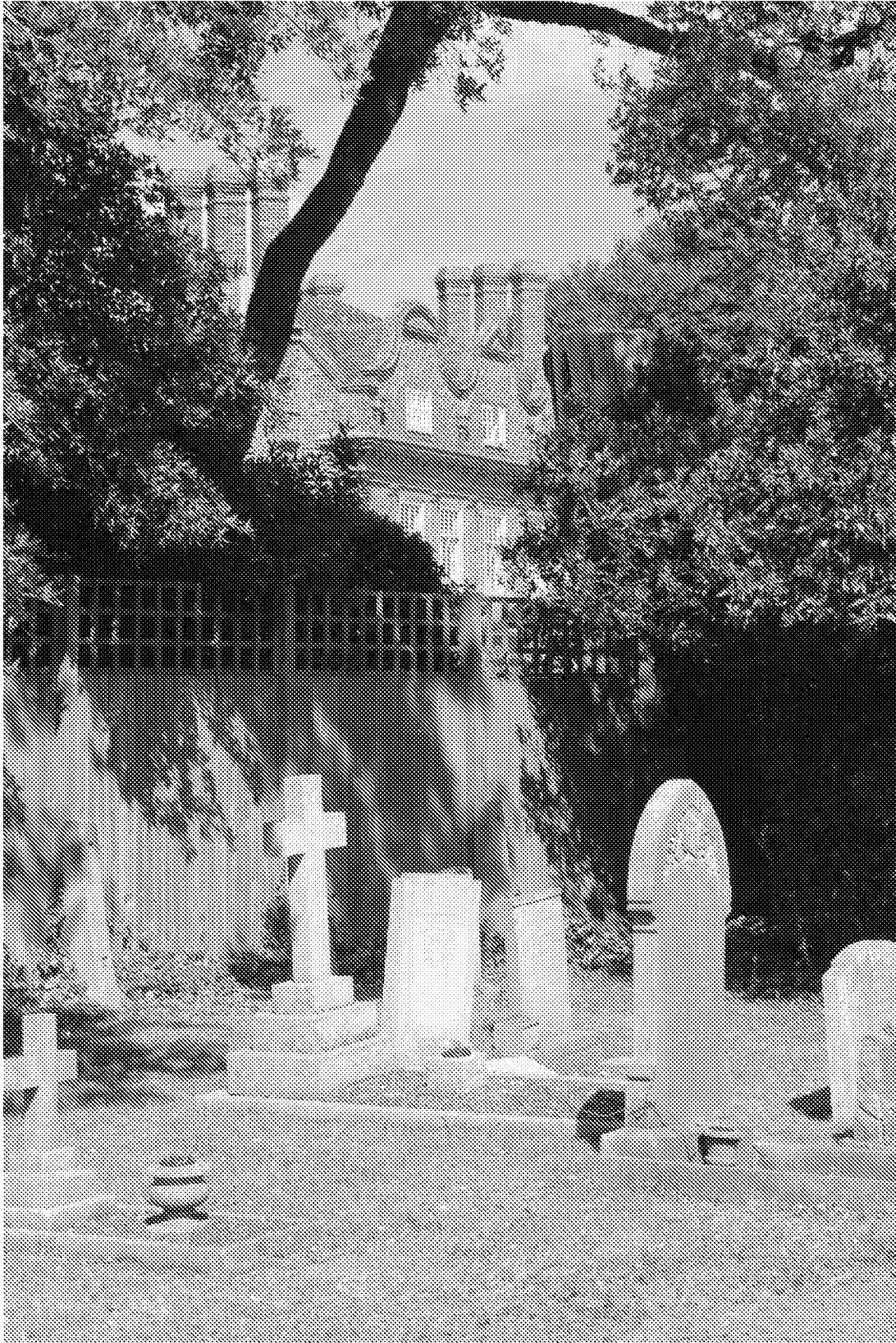
Image EDP 15: View of the Grade I listed Barnham Court looking north-west from within the churchyard and illustrating its close spatial relationship with the similarly Grade I listed parish church at the heart of the historic settlement core.
