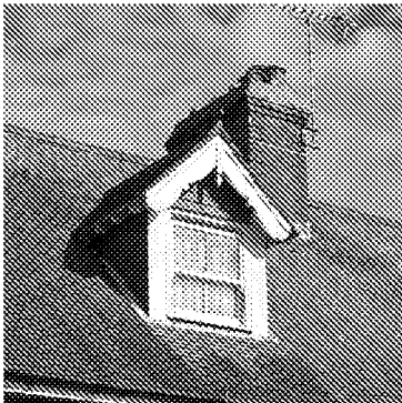
Pitched roof dormer
