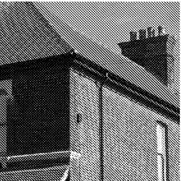
Black fascias and soffits
