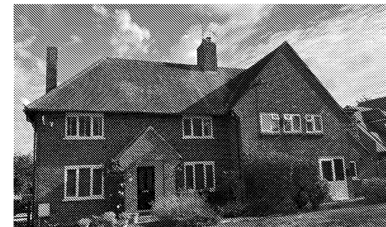
Hipped main roof with projecting gable and porch in Marshall Close
