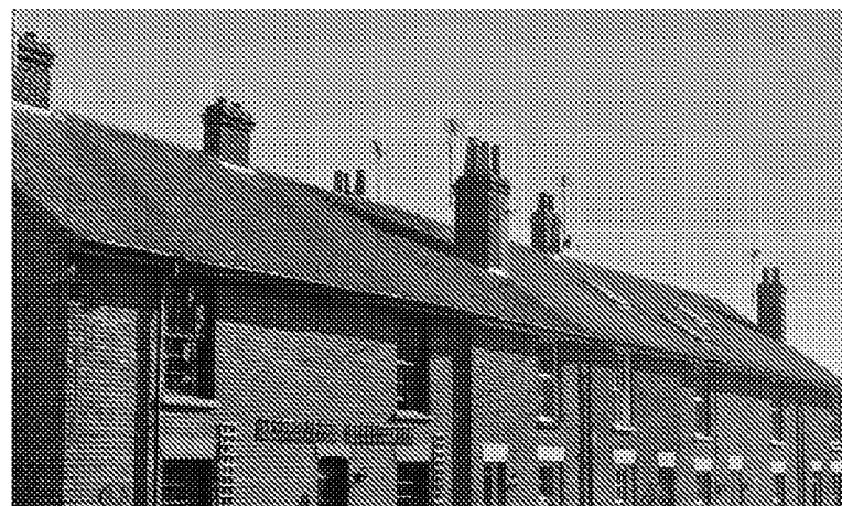
Multiple chimneys breaking up continuous roof line in Barnham Road
