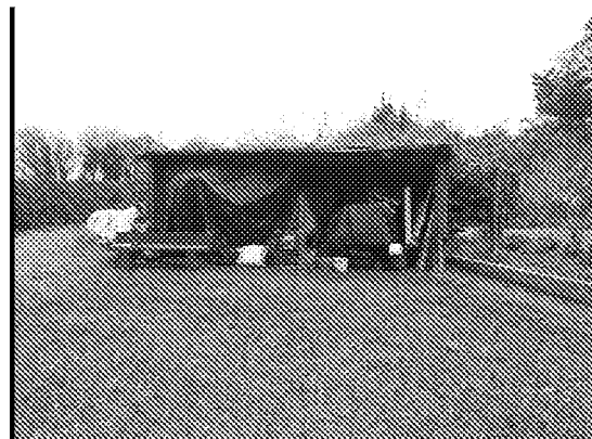
Existing agricultural structure
