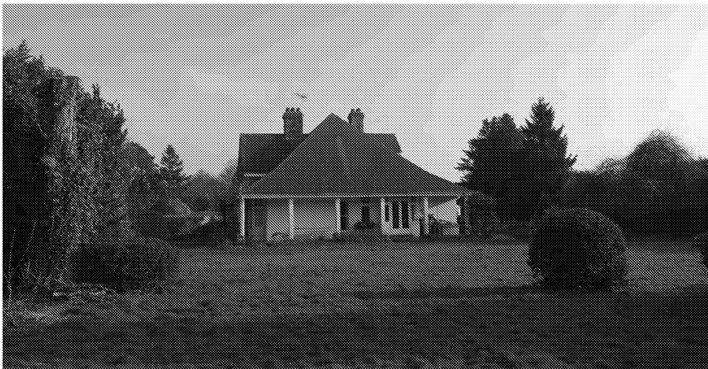
Photograph No. 1 - The amenity grassland garden with the dwelling in the rear.
