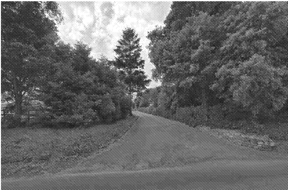
View of existing entrance into the site.
