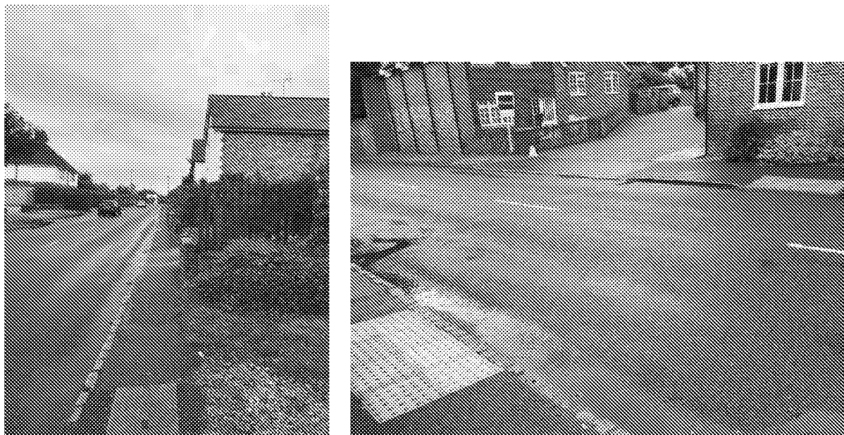
Photos 3.3 Footway East from the Application Site and the Uncontrolled Crossing Point
