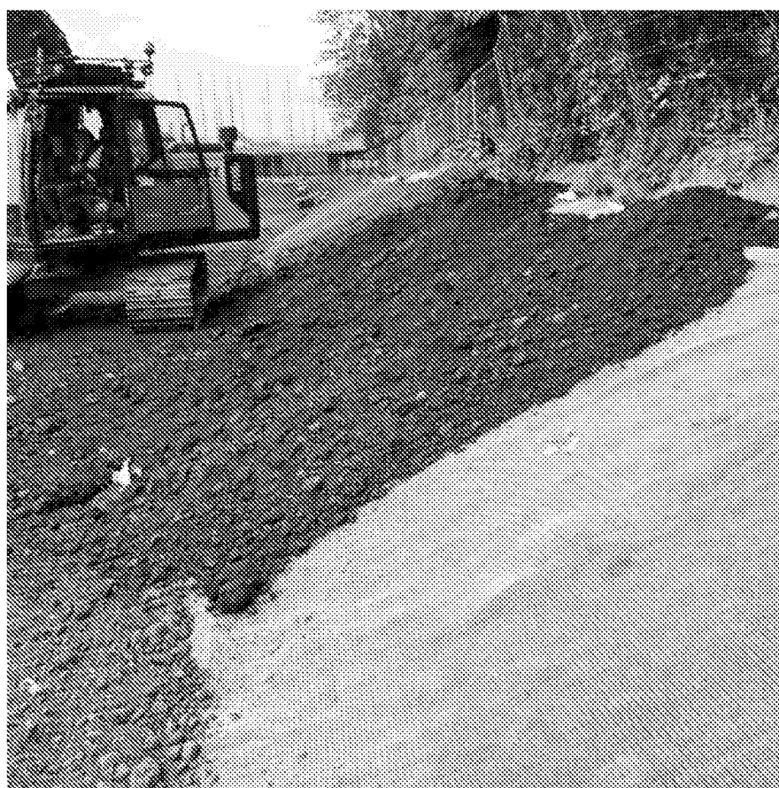
Photo 4 - Shaping southern bank to achieve 1 in 3 slope
