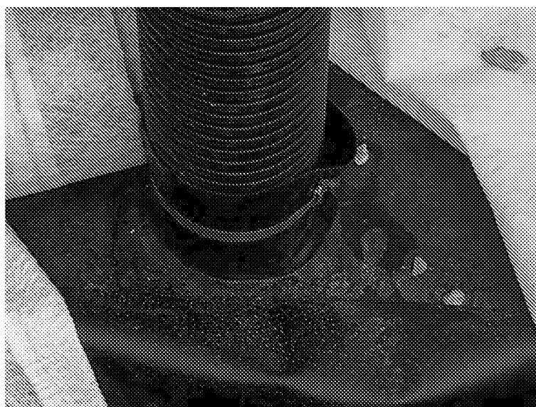
Photo 16 - Shows welded geo-membrane around air vent
