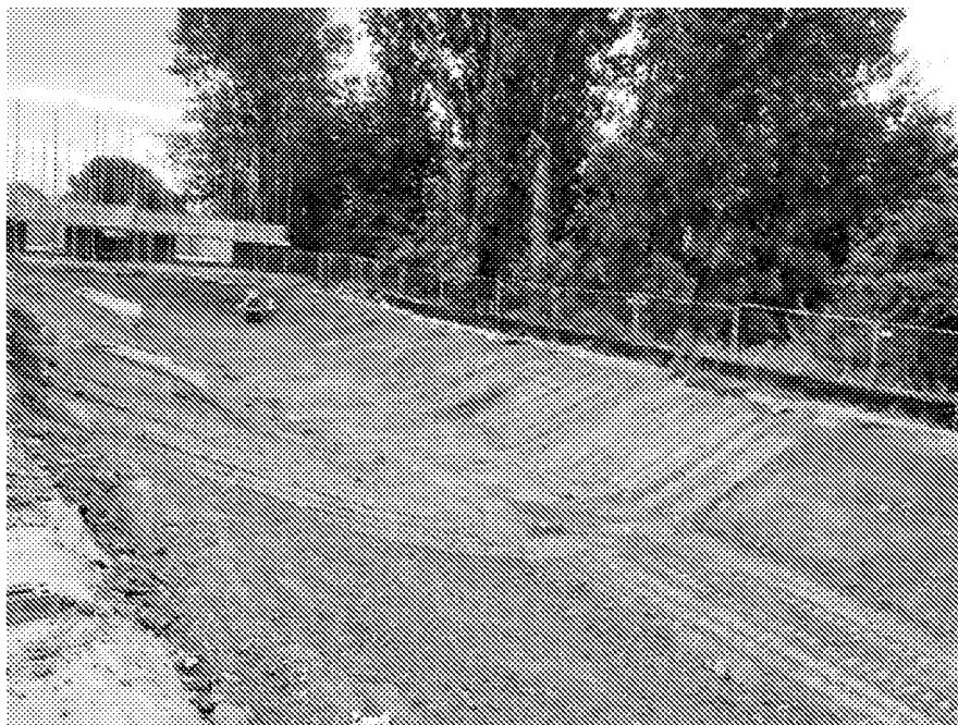
Photo 5 - Compaction of blue clay liner
