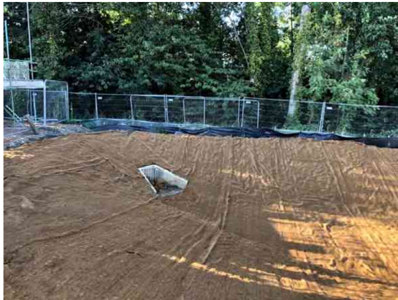
Photo 9 - Installation of bio-degradable erosion mat, east end looking at outfall
