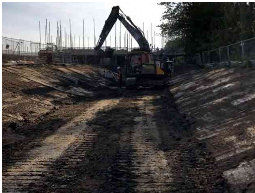
Photo 8 - Top soil layer looking east, trimmed and compacted
