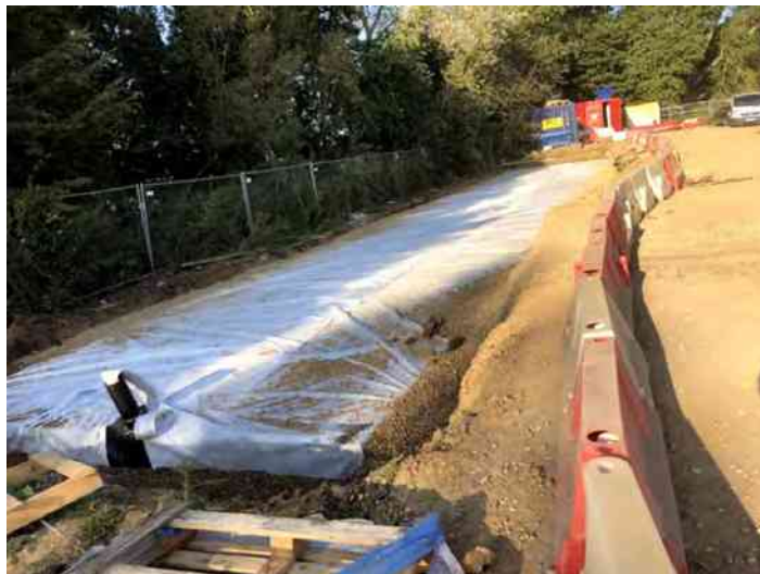
Photo 18- Backfill of attenuation tank looking west
