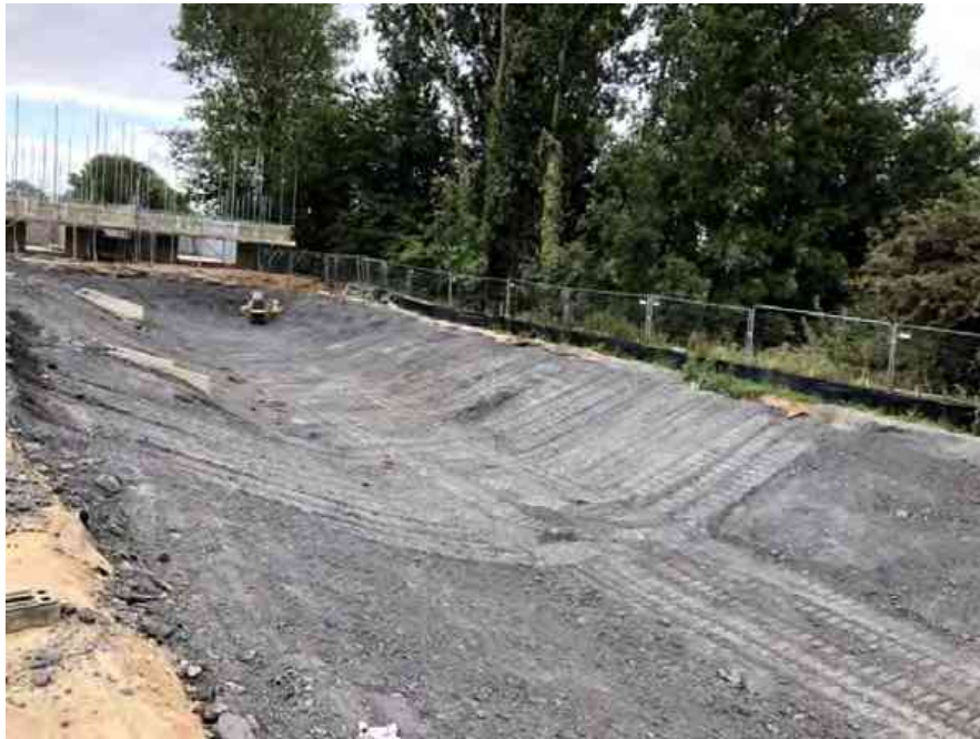
Photo 5 - Compaction of blue clay liner
