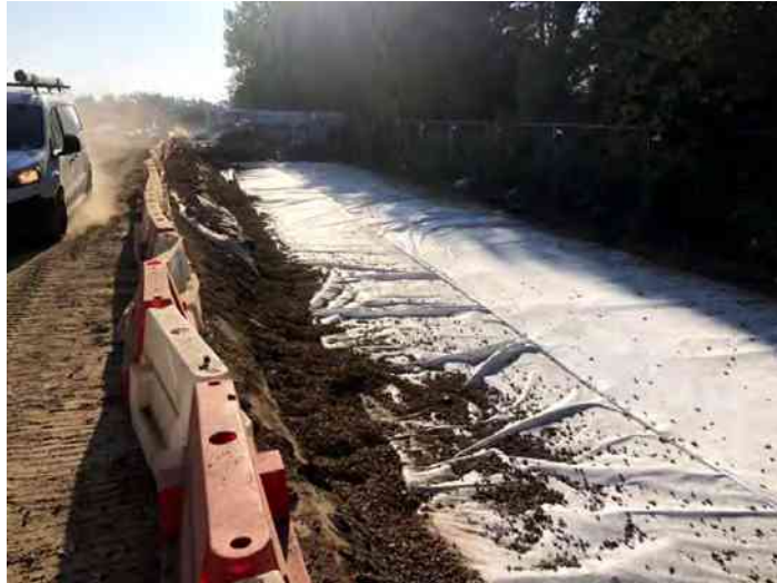
Photo 17 - Backfill of attenuation tank looking east
