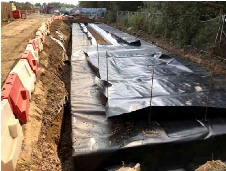
Box 13 - Shows central perforated pipe wrapped in geotextile back filled with fines free shingle crates both sides looking east
