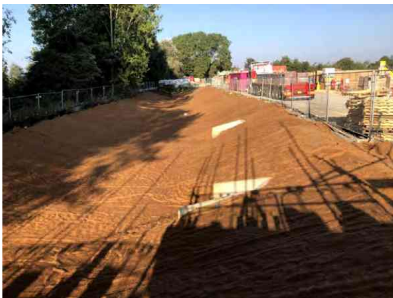
Photo 10 - Finished bio-degradable erosion mat looking west
