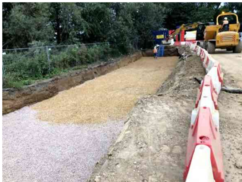
Photo 12 - Shingle base complete
