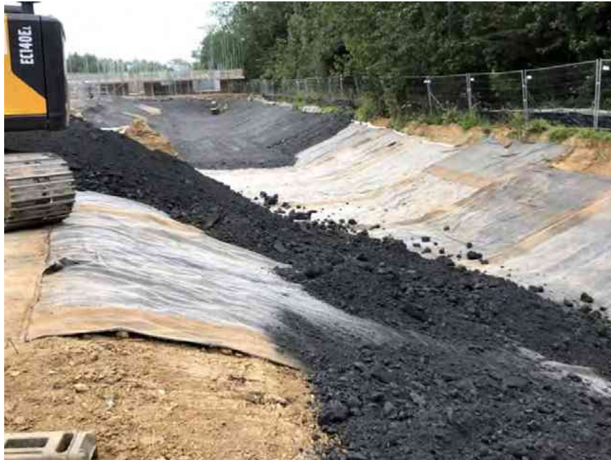
Photo 3 - Installation of bentonite liner and placement of blue clay pond liner
