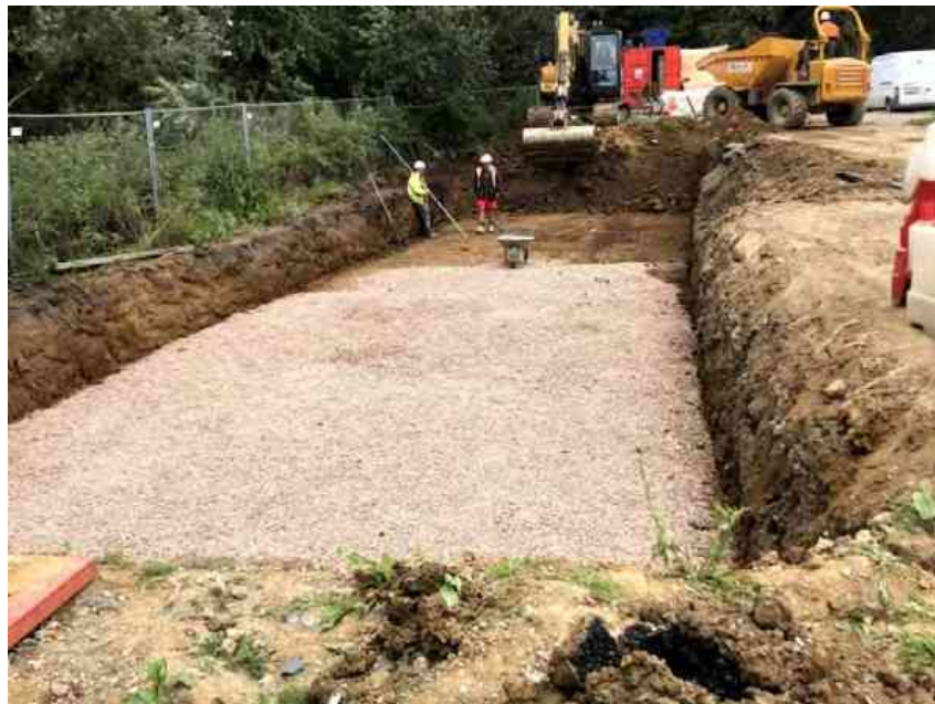
Photo 11 - Excavation for attenuation tank, note level control, and fines free shingle backfill
