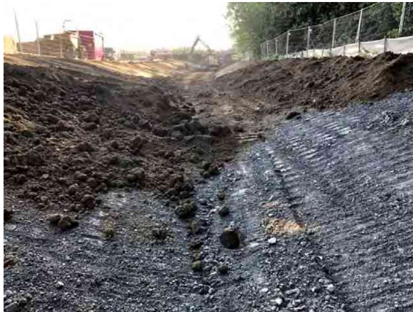
Photo 7 - Placing 150mm topsoil layer over clay
