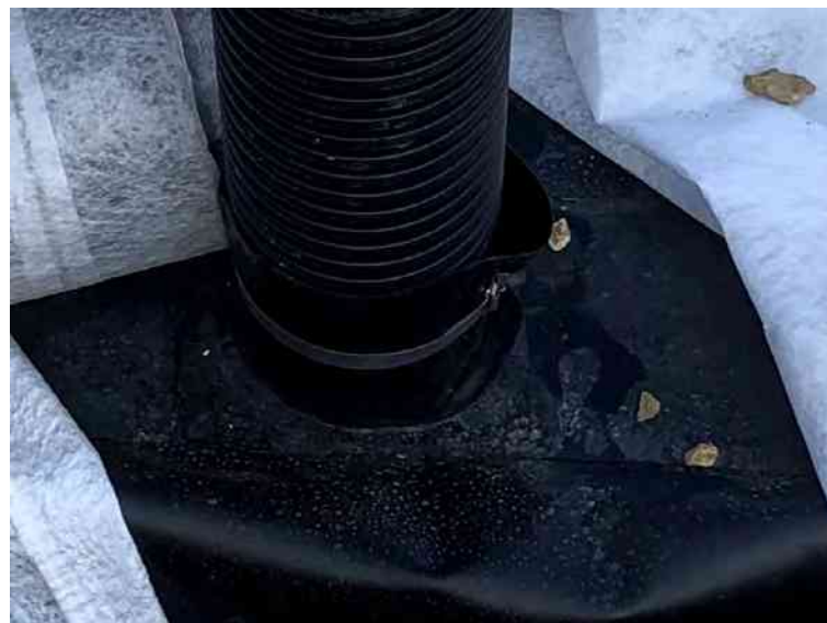
Photo 16 - Shows welded geo-membrane around air vent
