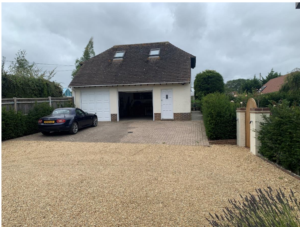
Photograph showing front of the existing annex & garage as shown from the driveway
