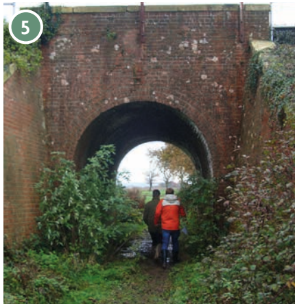
Pedestrian rail tunnel at the Rife Valley
