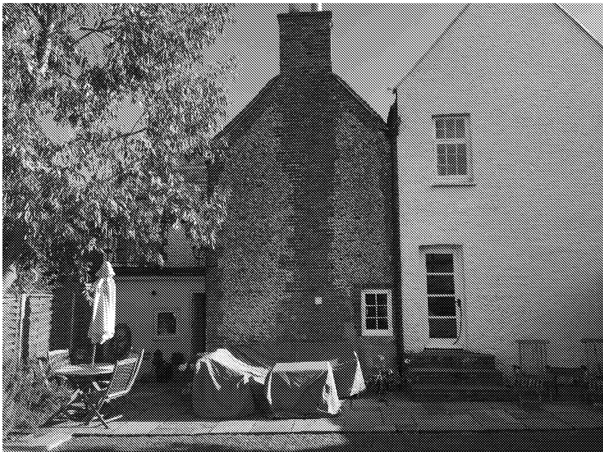
(Photograph 1 – Existing rear elevation viewed from the back garden)
