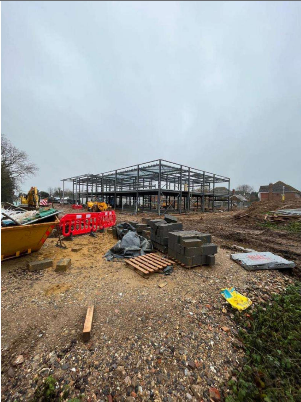
Photograph 2 – Active construction site to the south
