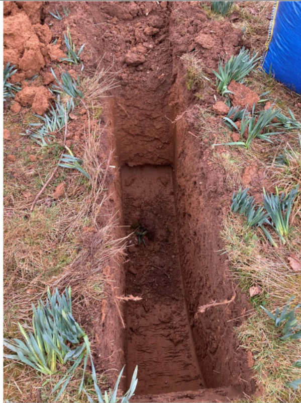
Photograph 7 – Pit horizons of SA202 prior to gravel soakaway cell installation
