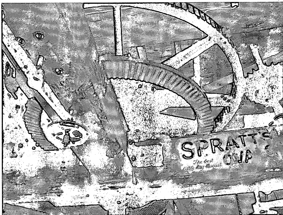
Cast iron spur wheels and tendering gear to be retained
