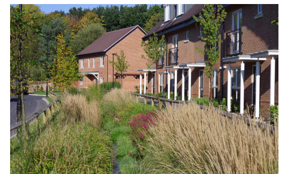
Vegetated swale integrated peri-urban streetscape
