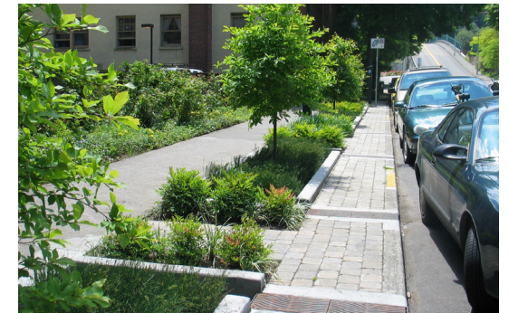
Urban canalised swales
