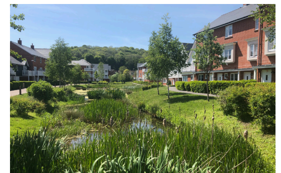
Vegetated swale integrated into semi-rural streetscape
