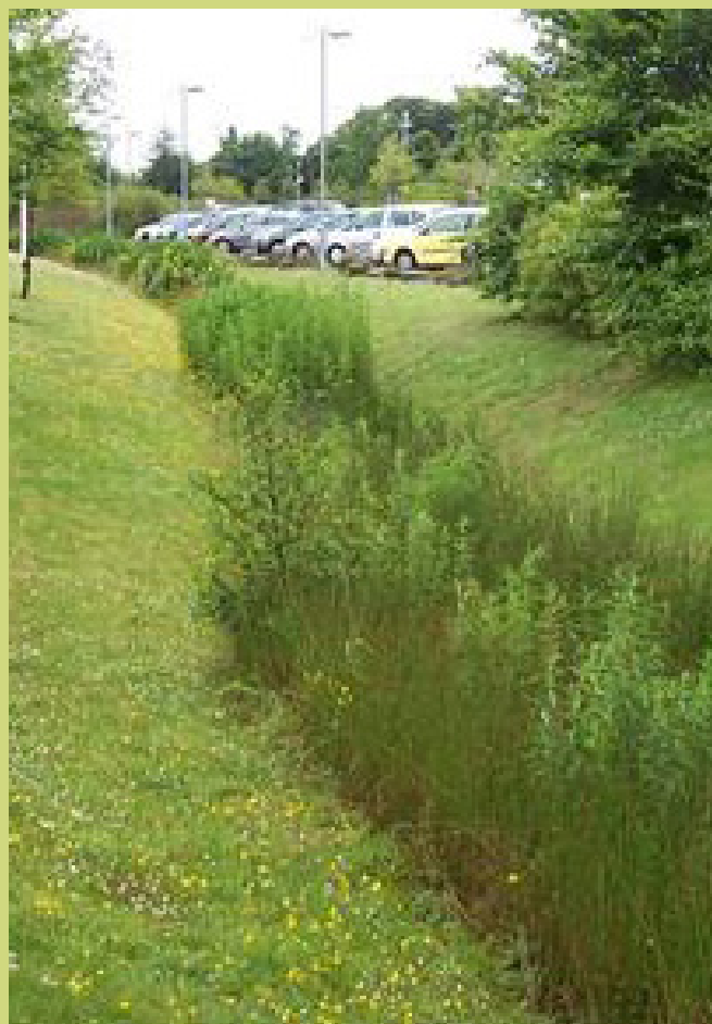
4. An example SuDS feature; swale
