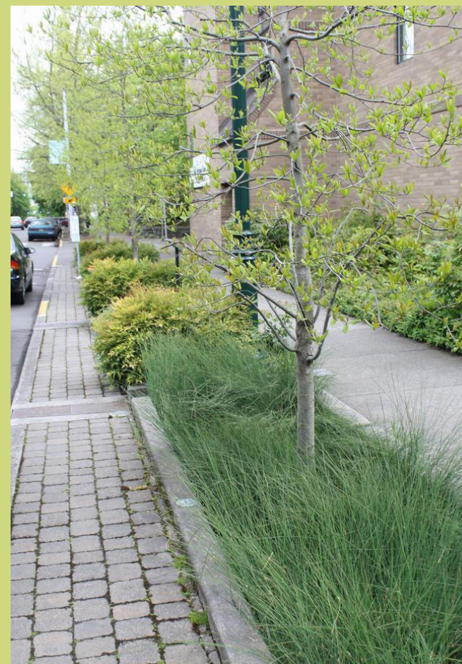
5. An example SuDS feature; roadside swale
