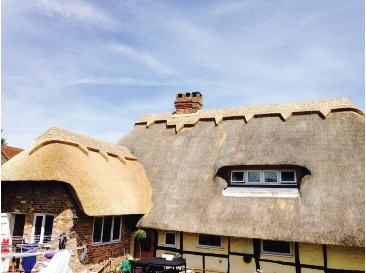
Extension is one coat of Combed Wheat Reed main house several coats of Combed Wheat Reed ( Tangmere)
