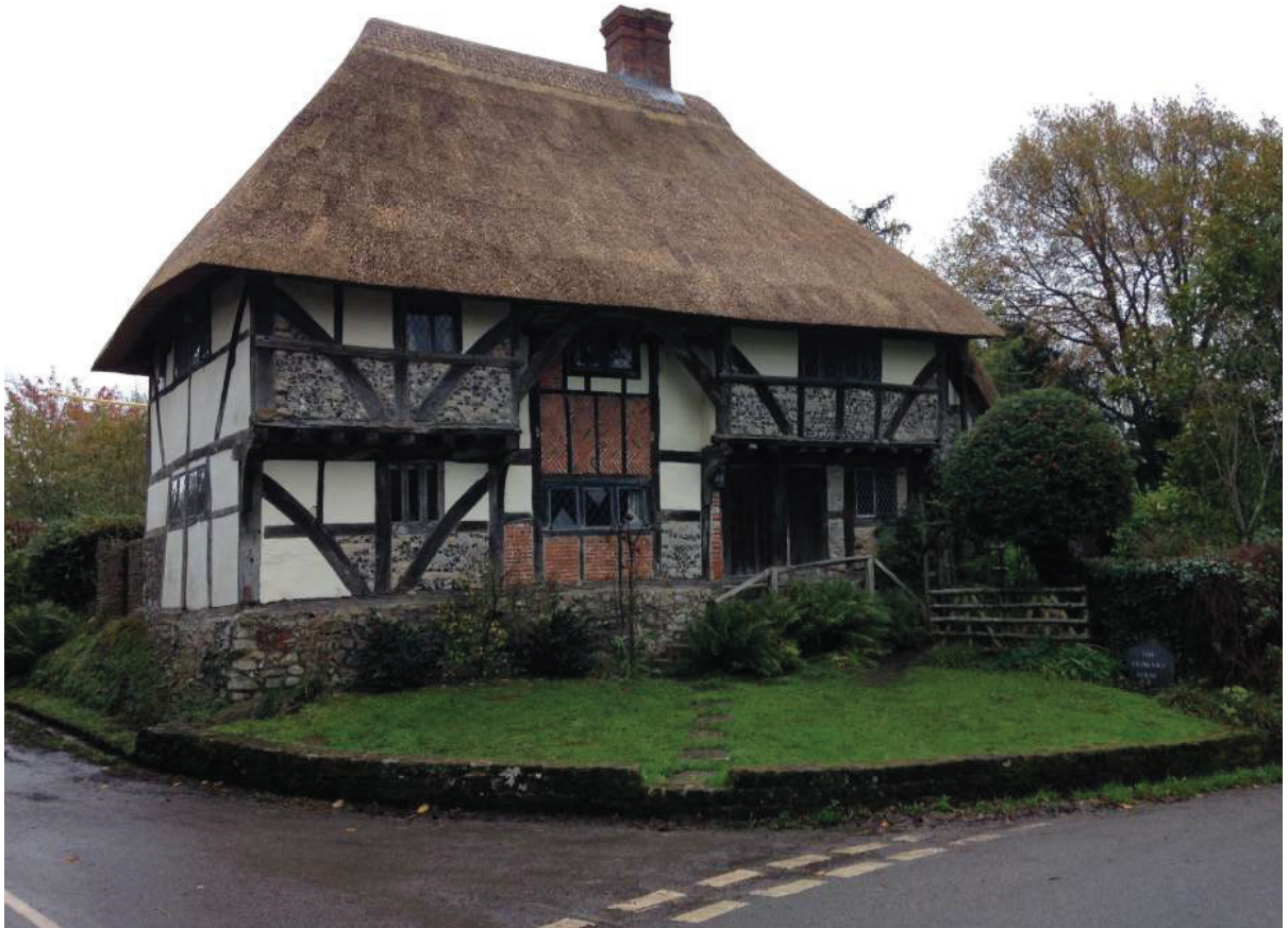
One coat of Water Reed , flush ridge (Yeomans Bignor )
