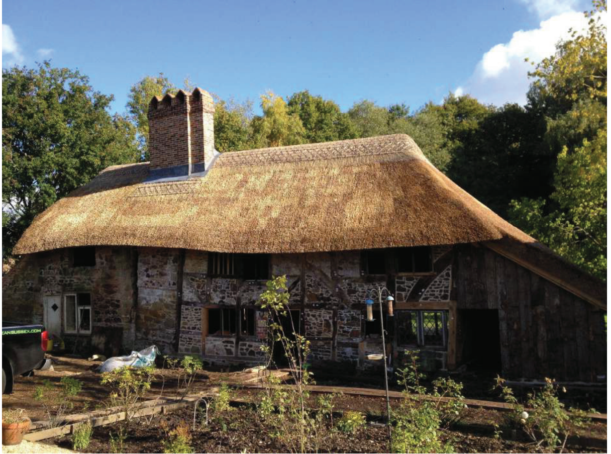
One coat of Water Reed with a traditional flush ridge, softened as much as possible with only one coat ( School Lane Fittleworth )
