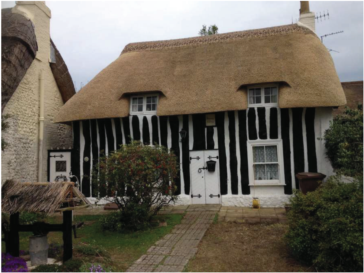
Combed Wheat Reed but many layers thick creating that fatter softer look. Note it is the many layers creating this look rather than the top layers type of thatch ( North Bersted Street Bognor Regis )
