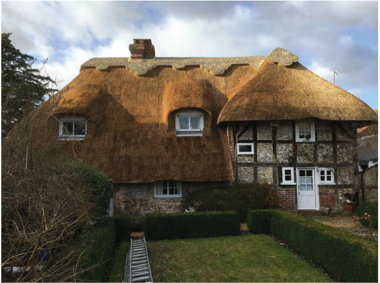
Several coats of old thatch with Water Reed on the surface ( Coates Cottage West Burton )
