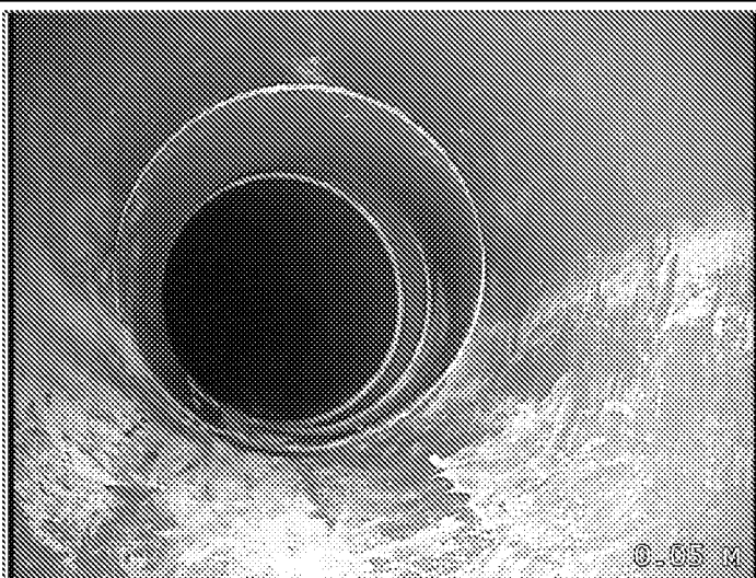
Start of Survey Length, Start node type, manhole, reference SW-200, Water level 0% height/diameter
