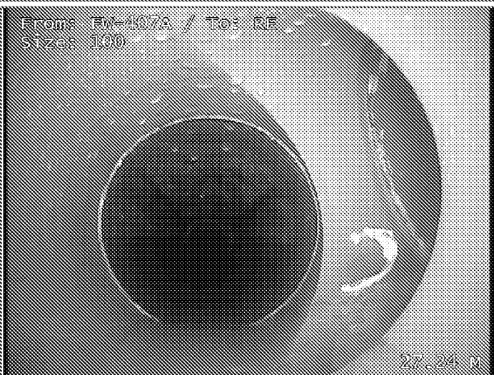
Junction at 1 o'clock, diameter 100mm
