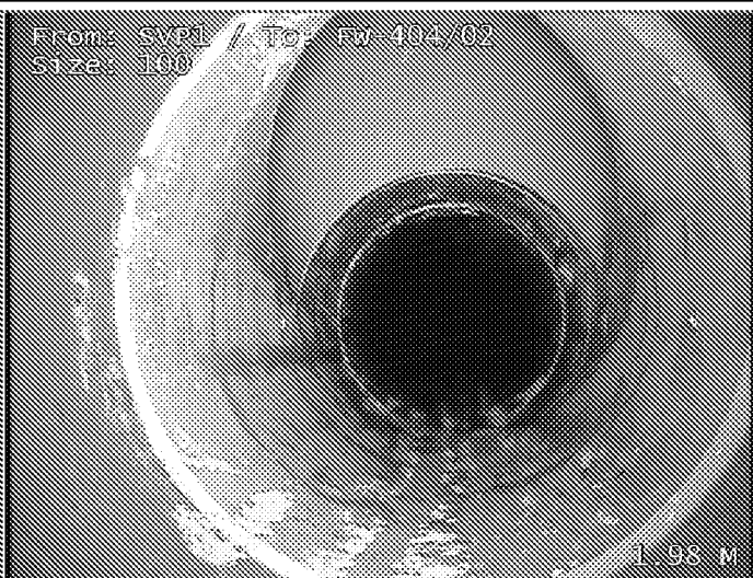
Junction at 12 o'clock, diameter 100mm - Remark: SVP2
