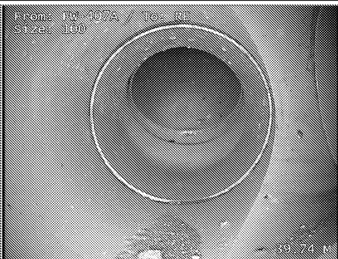
Junction at 1 o'clock, diameter 100mm
