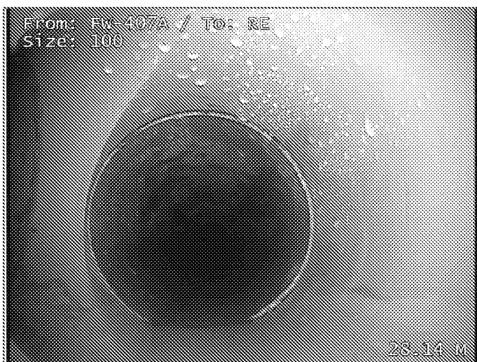
Junction at 10 o'clock, diameter 100mm
